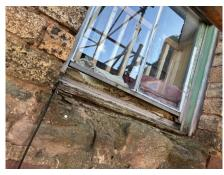
In lines with the general condition of the block, the windows throughout are in a poor and failing condition. Mostly are noted to be in a poor condition with minimum maintenance carried out to them over the years.
