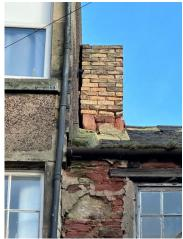
Due to ongoing recent water ingress problems, temporary repairs have been carried out by a roofer, the most recent carried out in December 2023. This was very much a temporary fix and as can be seen from this photograph of the rear there are a number of defects to the roof, chimney, gutter, windows and masonry areas that need immediate attention.
