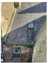
The slates to all roof slopes are in poor condition. They are thought to be a mixture of scotch and welsh (where a purple tint can be seen) and noted to be covered in moss, porous and likely nail sick. Due to the condition and size of these slates it is considered unlikely that many of them will be able to be saved and reused as the redressing of them will reduce their size further negating their use.
