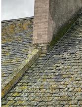
The stones to the existing skew copes are a mixture of stone to the front and concrete/aggregate to the rear main and lower slopes/pediment. The majority of skew copes to the rear are defective and beyond their life span.
