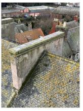
There are 2no chimneys to the property, one is mutual with no. 64 and one is a dwarf chimney sitting within the edge of the roof abutting the neighboring property on the other side. Both chimneys have lost their pots and the dwarf chimney has completely lost its cope, open areas have been patch repaired with slates to stop ongoing water ingress issues.
