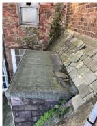
The only area of flat roof is the roof of the dormer to the rear. This is in poor condition and beyond its lifespan.
