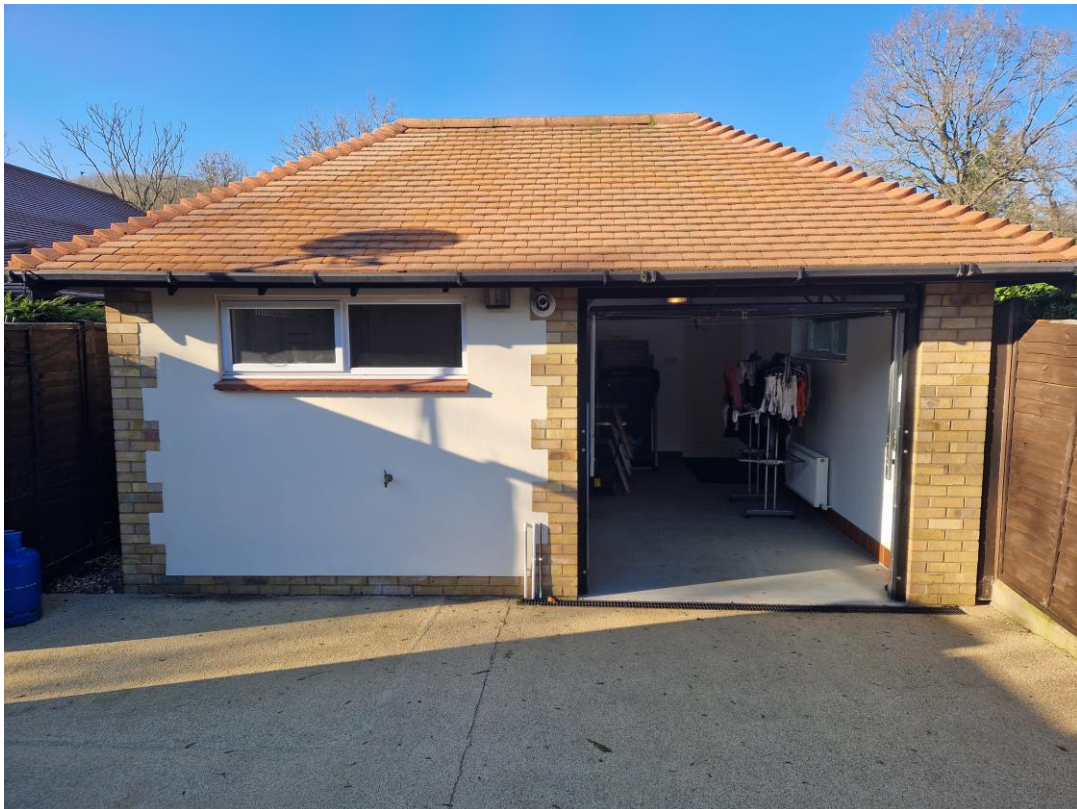
Rear View of Annexe Building.
