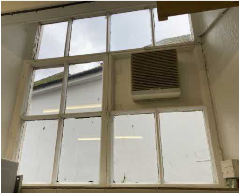
Fig 6 - Window W.3 - Inside View.
