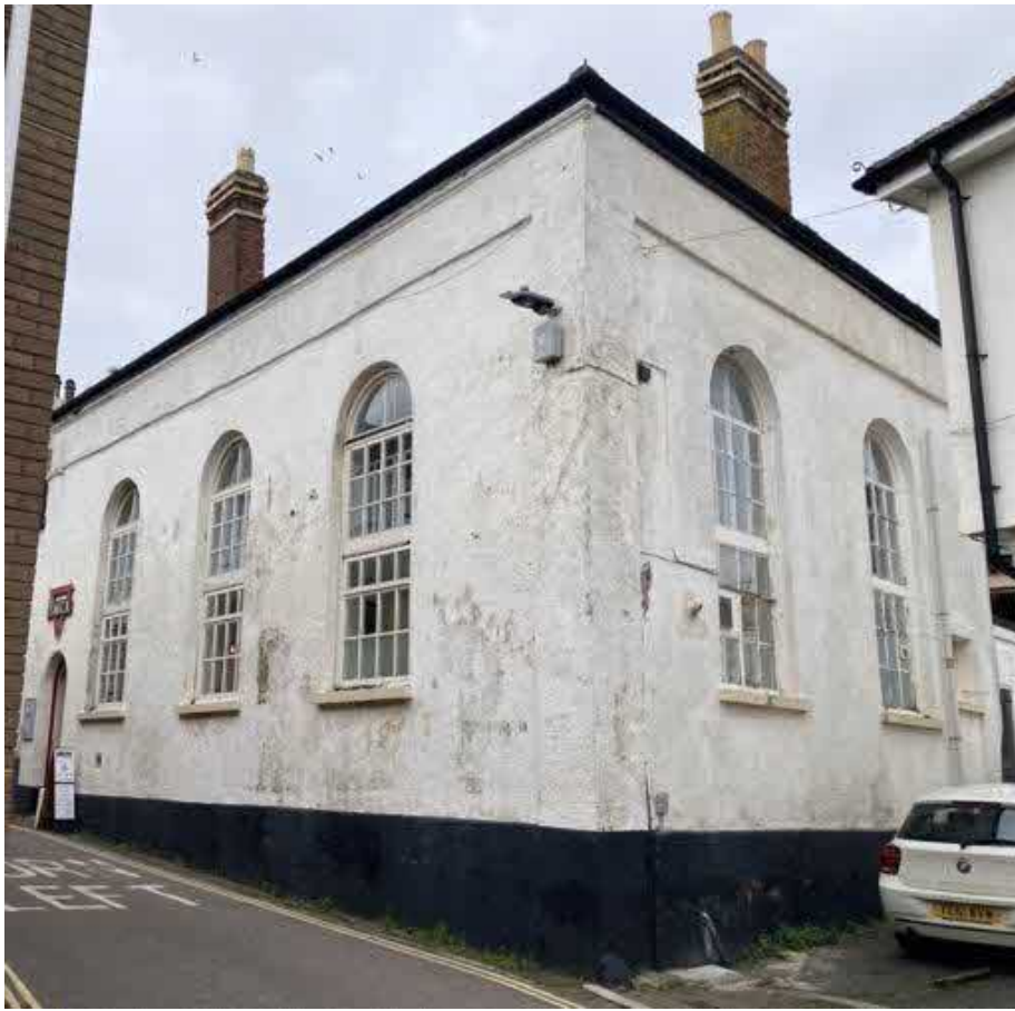
Fig 1 - Two Main External Elevations.
