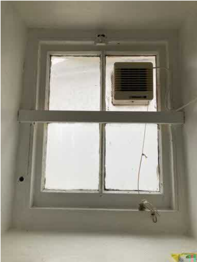
Fig 3 - Window W.1 - Inside View.
