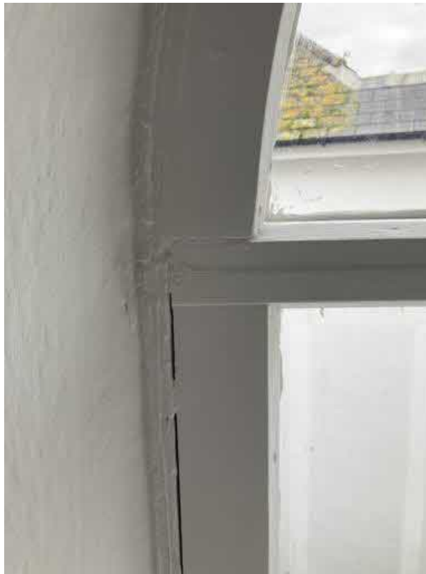
Fig 14 - Window W.7. - LH side (Inside).
