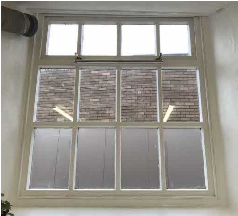
Fig 9 - Window W.4. Inside View.
