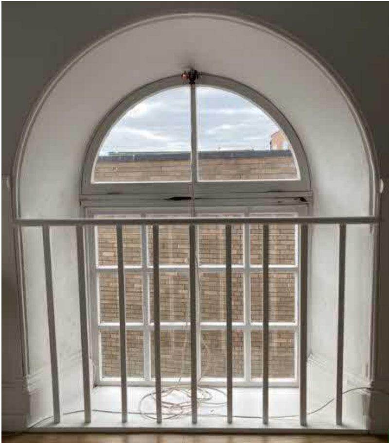
Fig 8 - Window W.9. Inside View.
