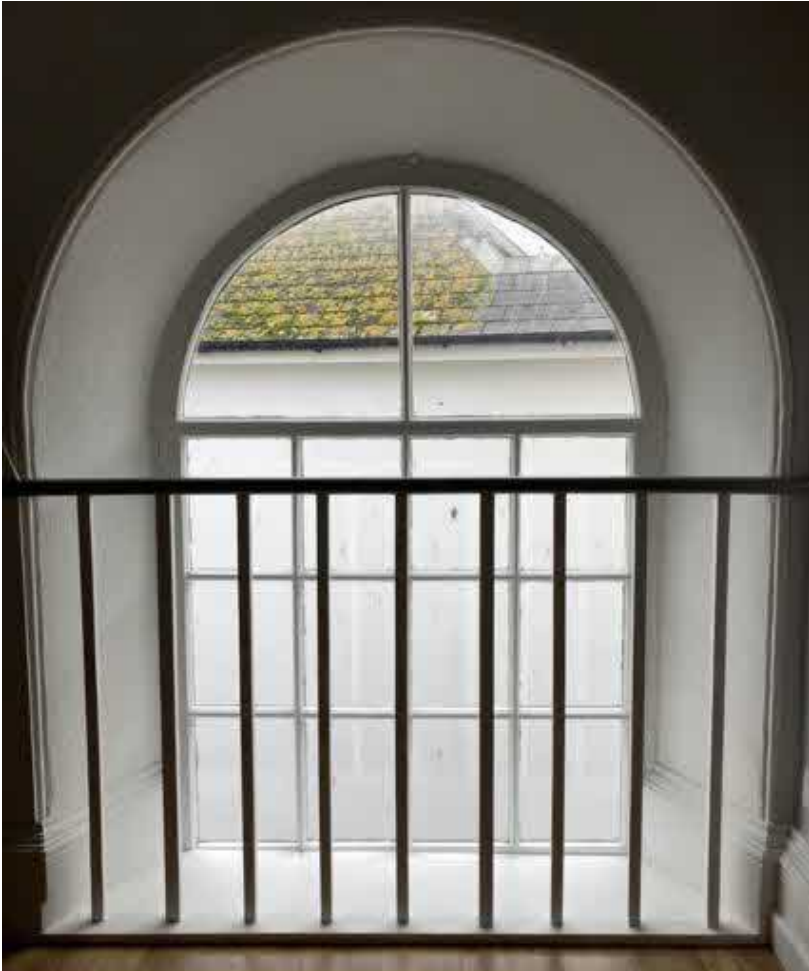
Fig 5 - Window W.7. - Inside View.
