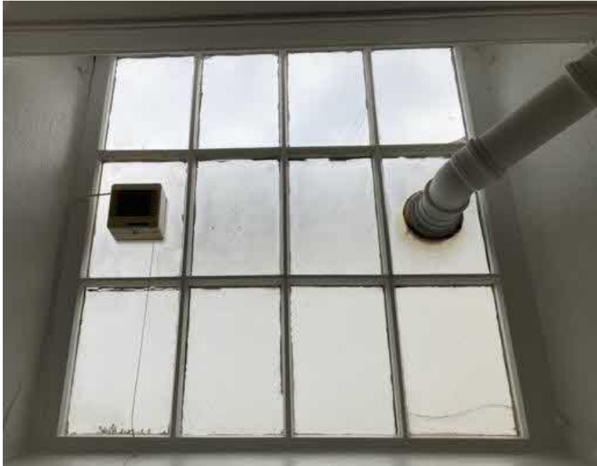
Fig 4 - Window W.2. - Inside View.
