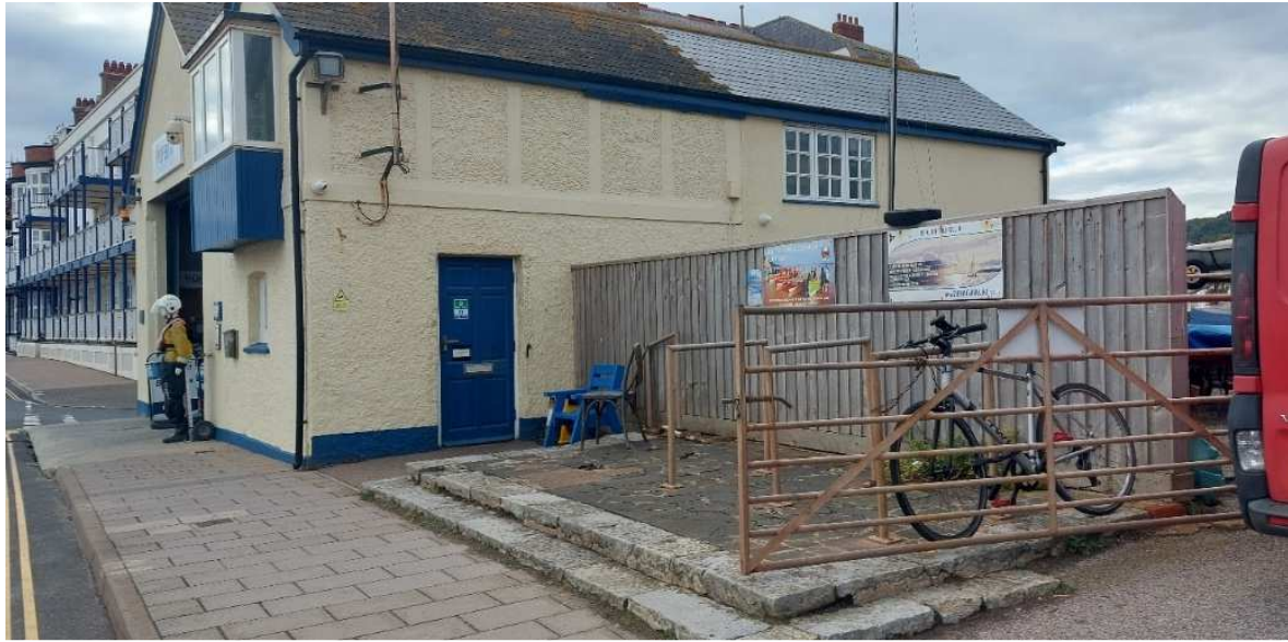
Figure 19. Location of proposed extension. Photo by Studio Four Architects
