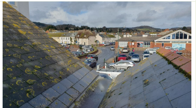
Tight roof slates and ridge tiles
