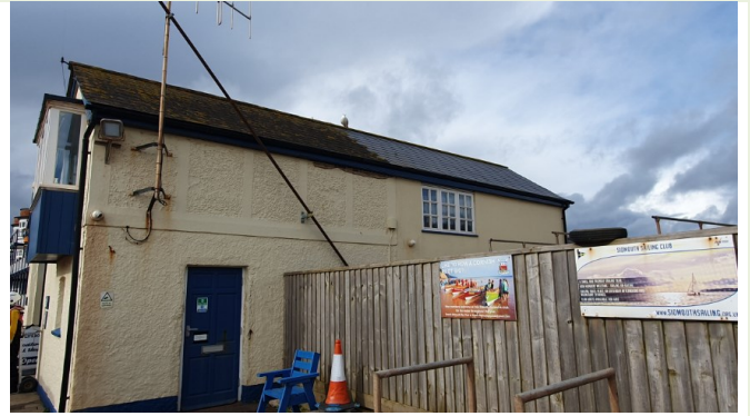
Eastern elevation – office structure
