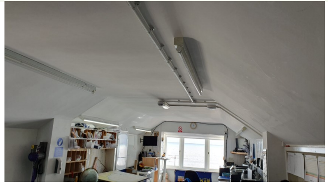
Vaulted ceiling of office structure
