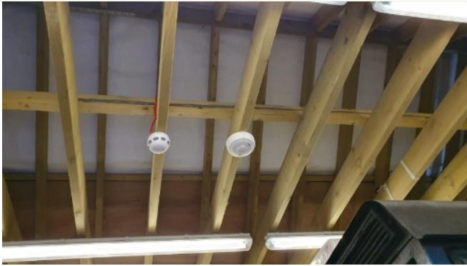
Internal roof of rear garage
