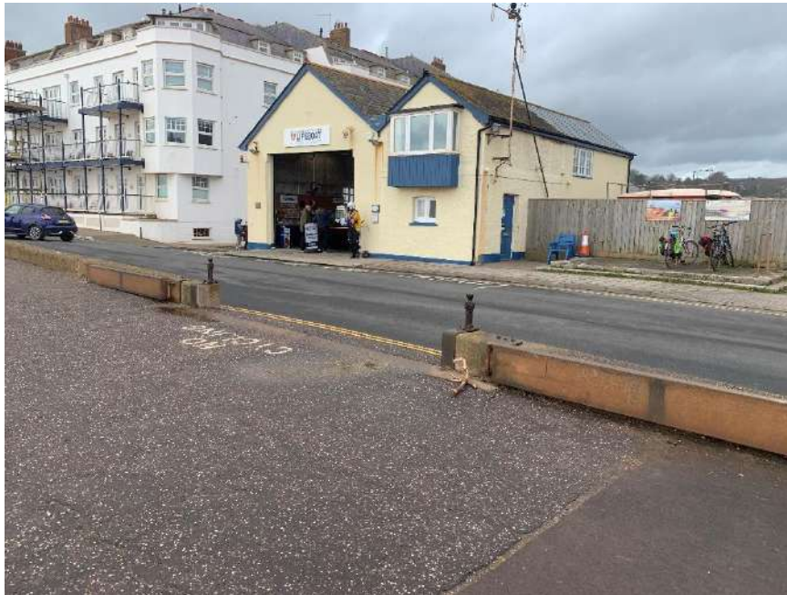
Photo 1. External view of existing lifeboat station, proposed development site to the right of the picture
