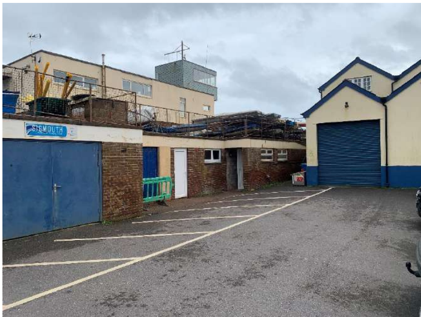
Photo 4. View from lower-lying ground to the north, facing south towards the proposed extension location.
