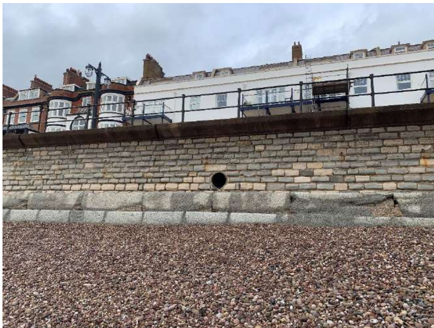
Photo 10. Surface water outfall from The Esplanade to the beachfront
