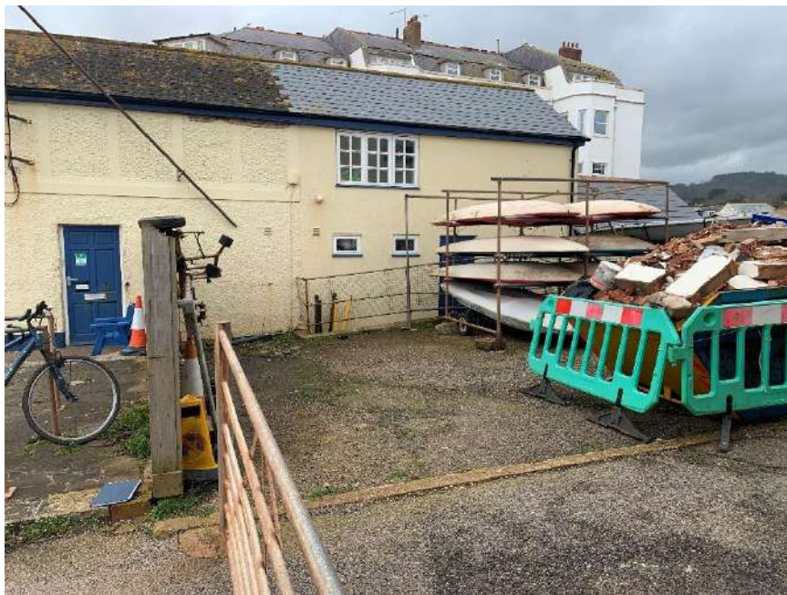
Photo 2. Proposed development site currently in use for boat storage
