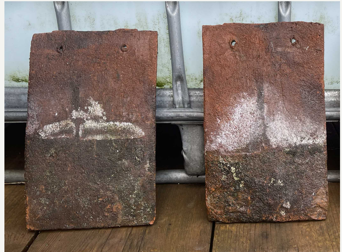
SPARSHOLT MANOR MAIN HOUSE EXISTING ROOF TILE
