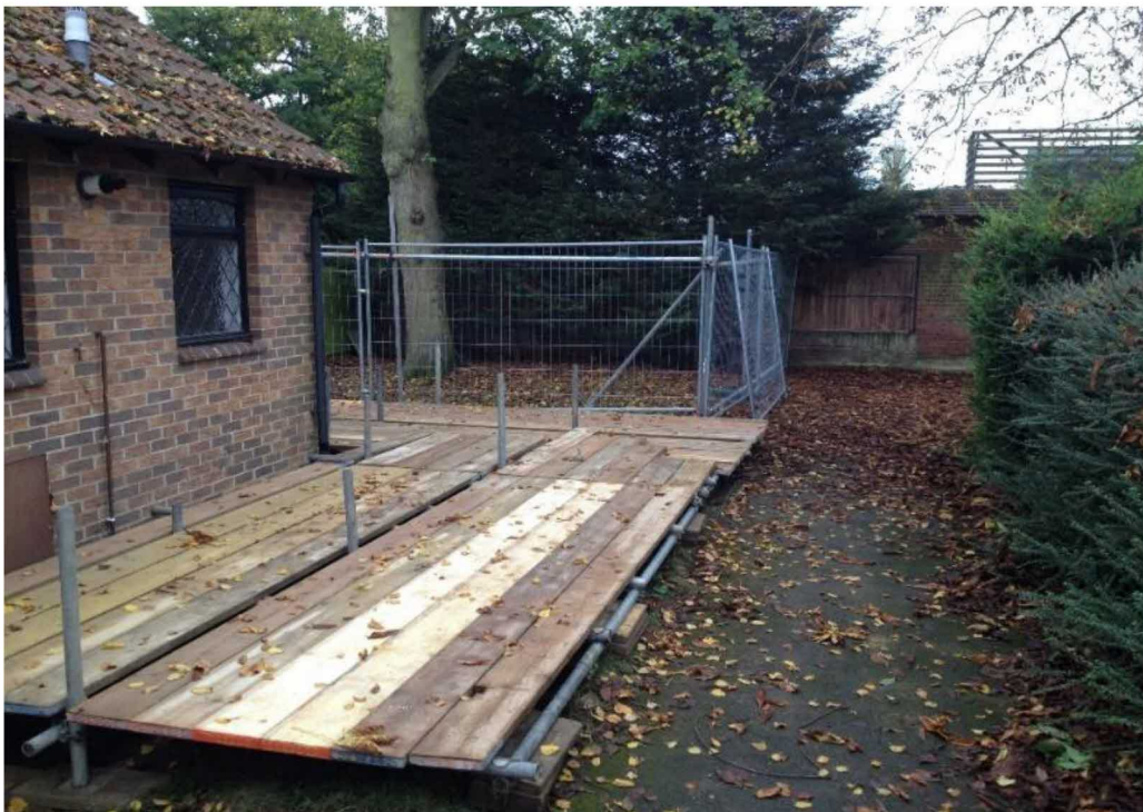
Figure 7 – Specification for scaffold ground protection.
