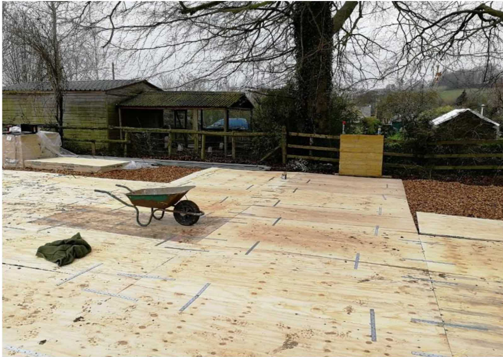
Figure 6 – Plywood sheeting used as ground protection.
