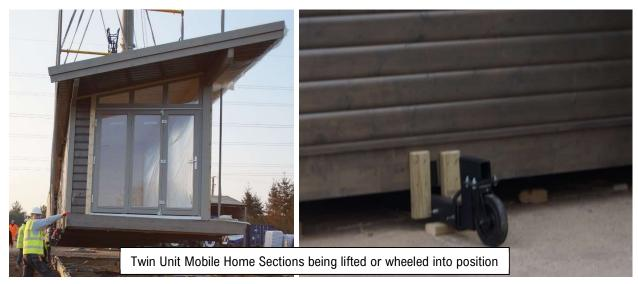
Due to the size of the proposed twin unit caravan, the road and site access complexities, independent assembly of the two individual sections will take place on site, they will then be moved into position with connecting as the final act.
