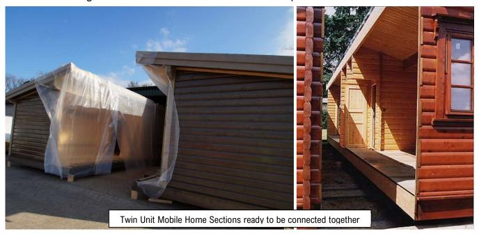
The process of assembly is identical whether undertaken offsite or onsite. The two sections of a twin unit caravan are independently assembled, they are then brought together by lifting or wheeling into position (see below), with the final act being connection of the two sections to form a whole.
