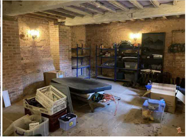
Ground floor store at south end of building
