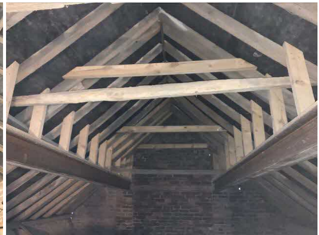
Roof over south end of building
