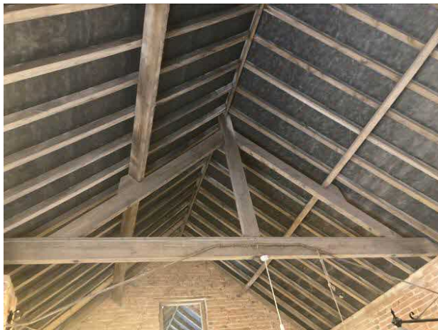
Underside of roof main storage room
