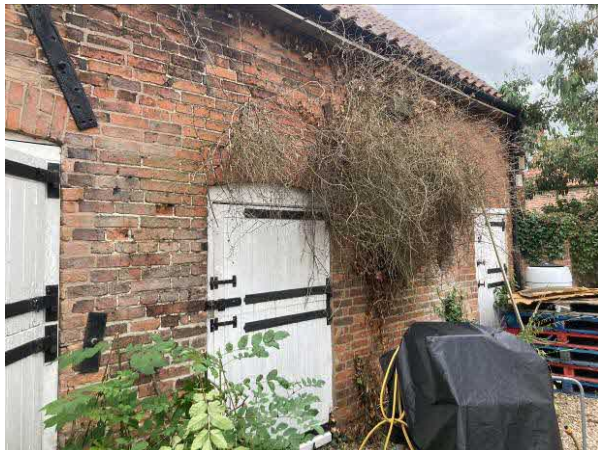
View of doors along west side
