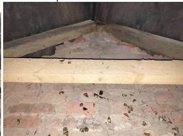
Feeding debris 13 September
