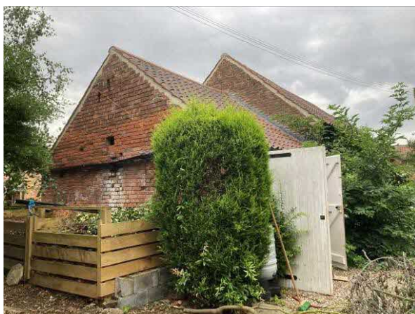
North gable end of building
