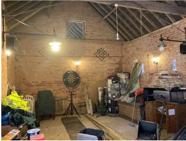
Main central storage room
