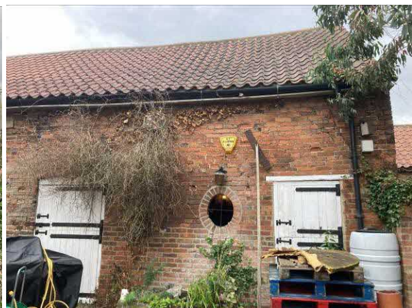
South end of building
