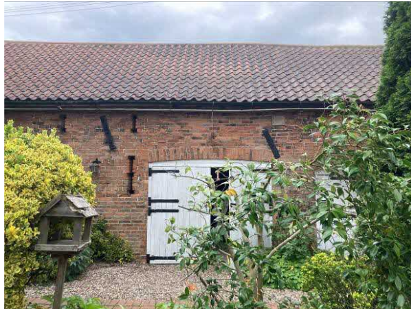
Centre of western side
