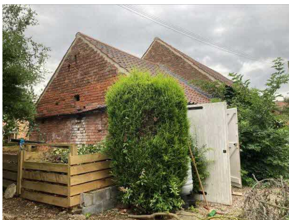
North gable end of building
