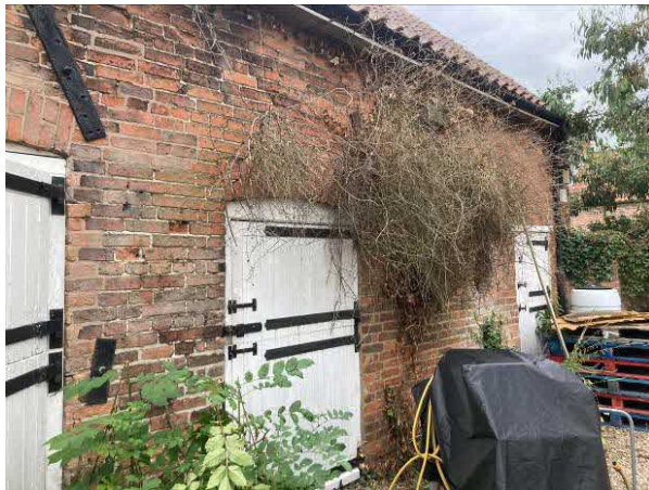
View of doors along west side
