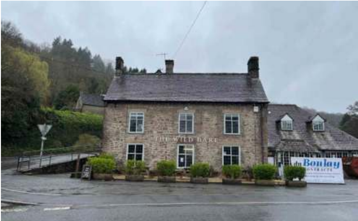
View from outside the site, looking toward The Wild Hare from the SW.
