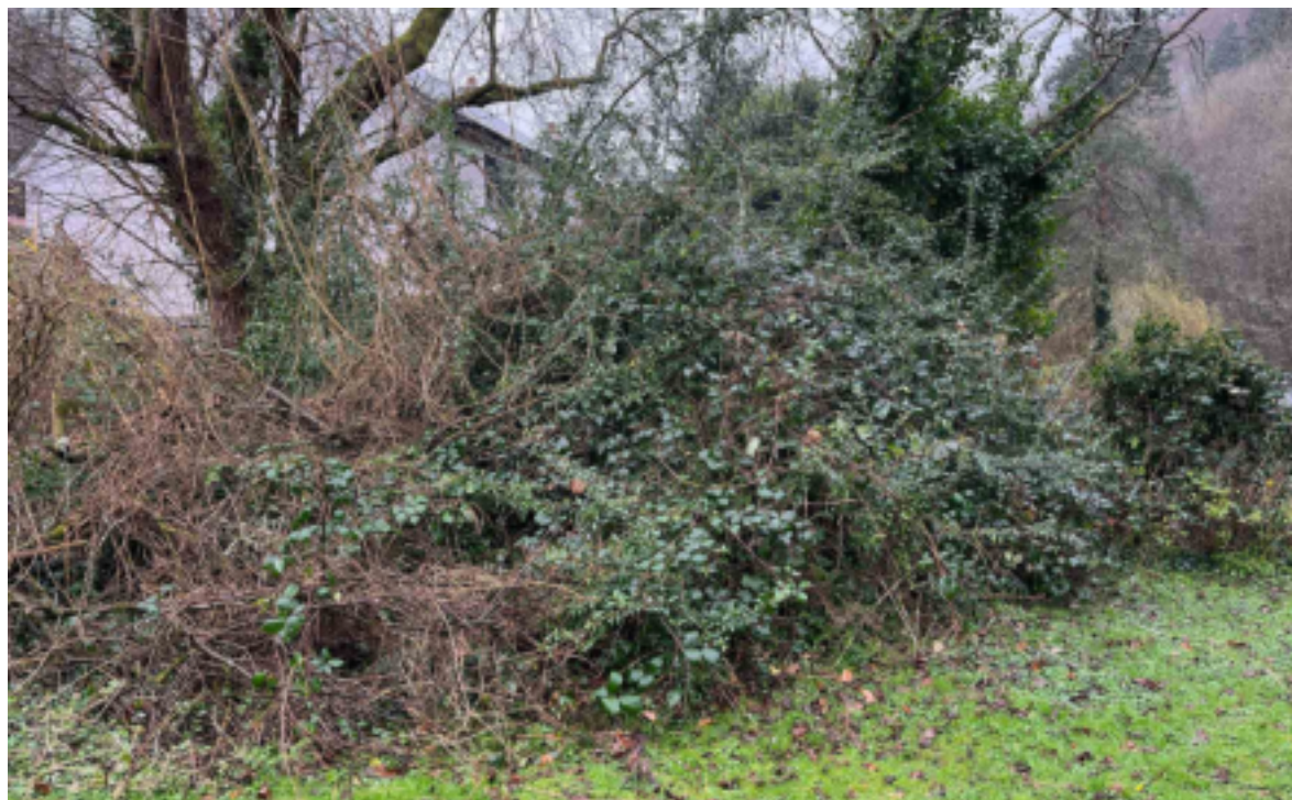
View from inside the site, looking at the side & rear of properties adjacent to northern boundary.
