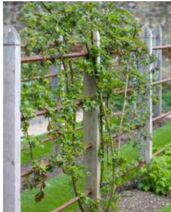
Carved oak posts and square section metal bars on the diagonal are used to create a division and plant support between the fine dining and the larger garden
