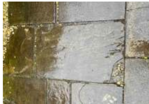
Existing stone slabs to be lifted and relaid where required.
