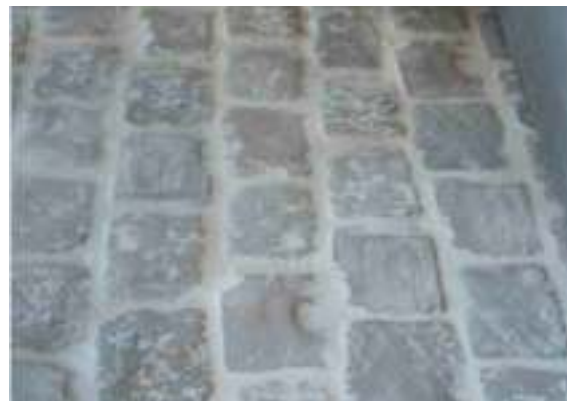
Concrete paver Terpstra from RAW stone - in an effective cobblestone size of 120 x 200mm will form the path at the cafe - matching the interior flooring
