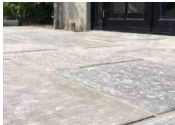
'Abbey Exterior' is a 22mm thick concrete paver from RAW stone which will be used for the fine dining terrace and the paths adjacent to the accommodation buildings. Offered in a subtle range of colours and natural stone finish, it is an attractive and economic surface which blends well with the Monmouthshire stone
