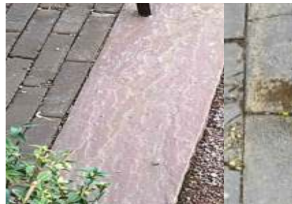
A natural pink sandstone laid as a 300mm wide flat edging or turned on it's side to form an upstanding edging between soil and hard paving or chippings.
