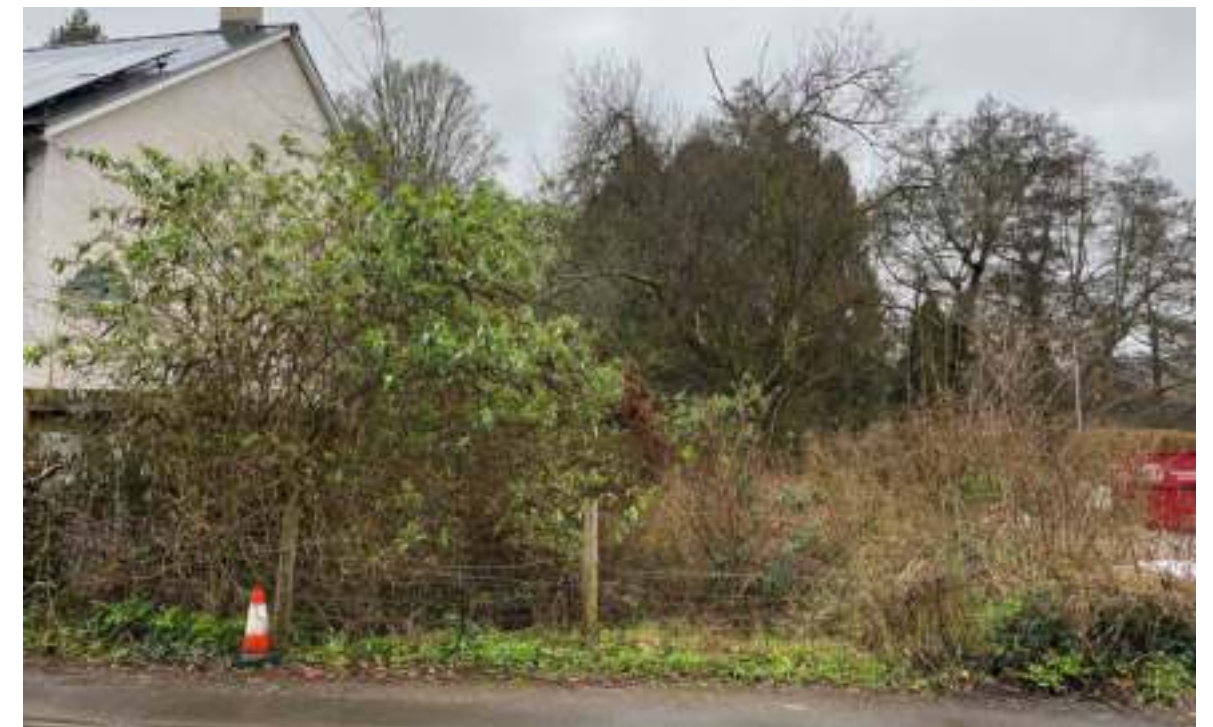
View from outside the site, looking toward the accommodation block over the existing car park clipped evergreen hedge (northern section).
