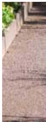
Local pink crushed natural stone 5mm to dust forms a well consolidated porous pedestrian surface of local character.
