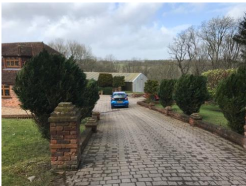
Photograph 5: Paving to east of B1
