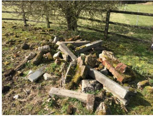
Photograph 8: Rubble pile within central fenced area (TN1)
