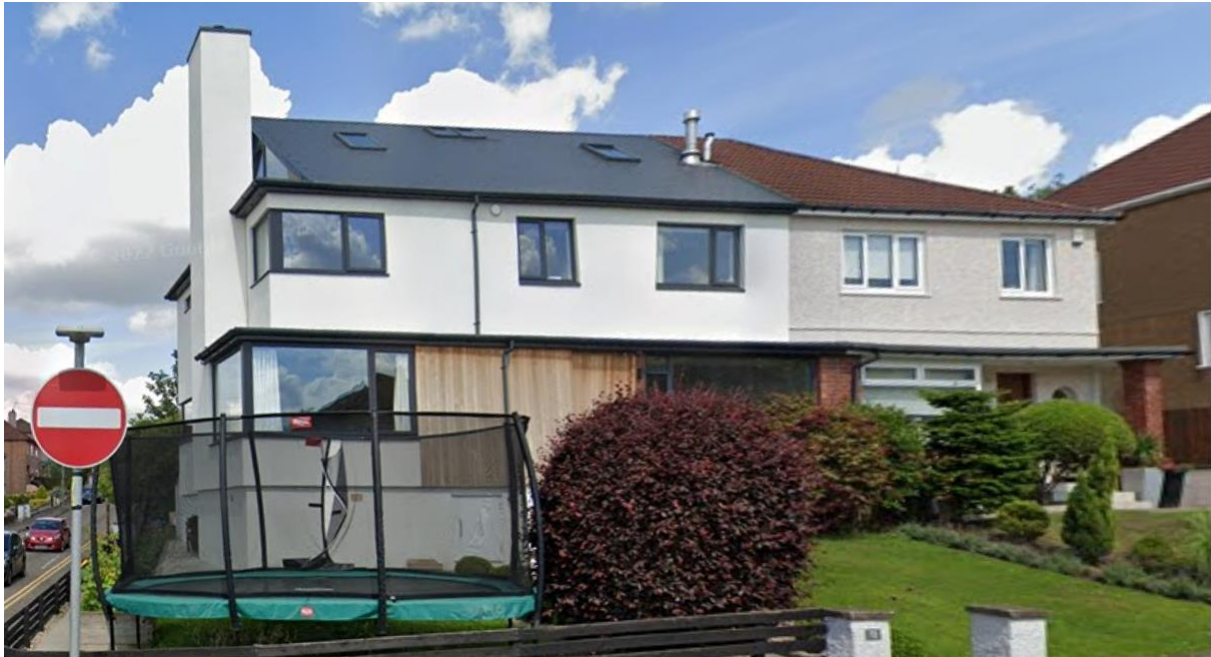
A recent extension in Whittinghame Drive
