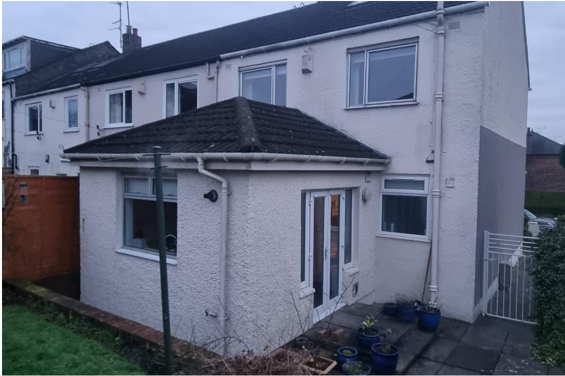
The terrace of 76 Mitre Road from the rear
