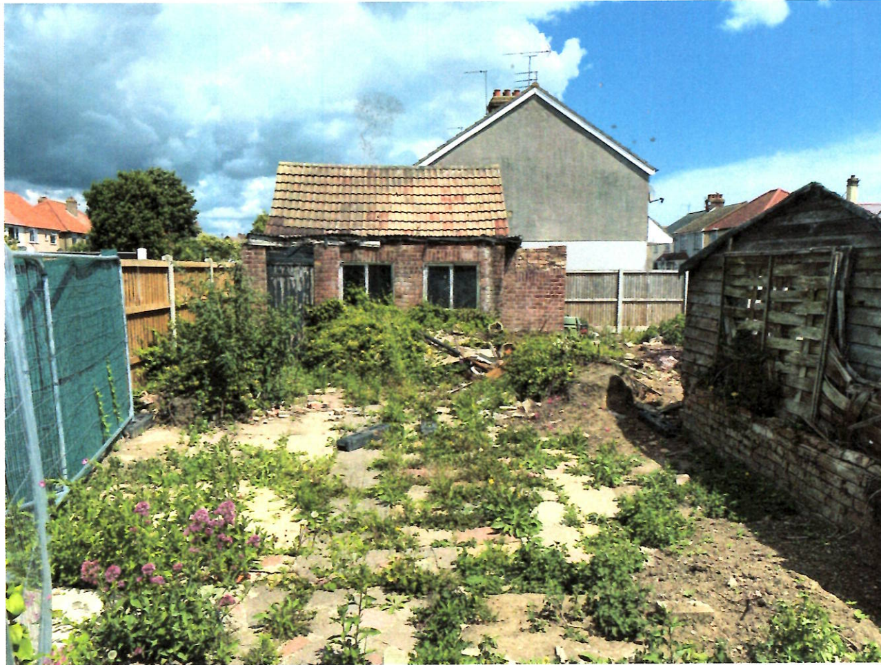
INTERNAL SITE VIEW NORTH EASTWARDS TOWARDS THE REAR BOUNDARY OF THE HOST DWELLING No. 152. OSYTH ROAD SHOWING THE EXISTING GARAGE BUILDING.
