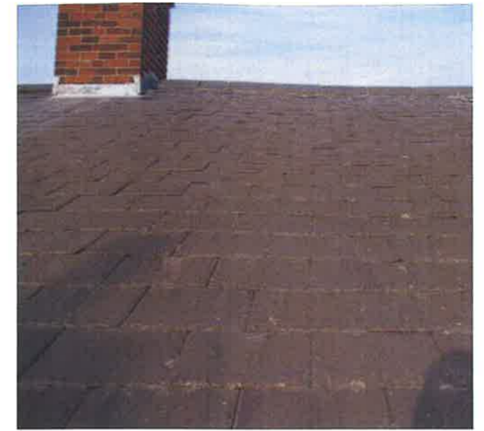
02 / 03 / 05 Roof covering / flashings /brickwork
