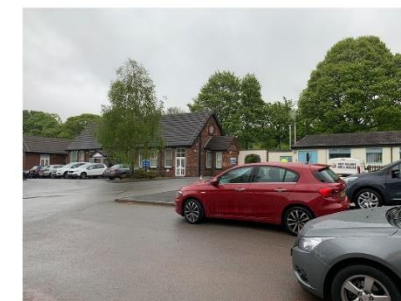
7. Scott House and Tredgold House
