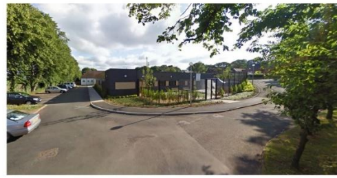
1. MacArthur Centre from Site Egress
