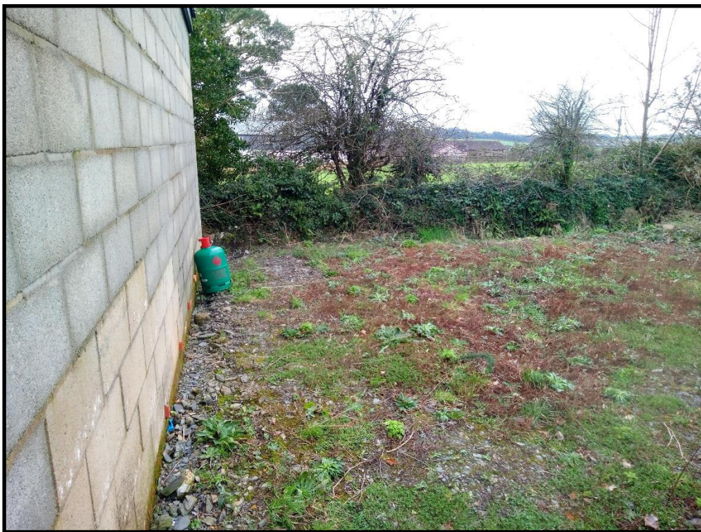
Photograph 8 – Photo of the rear of the garage in the southwest corner of the site. Empty and sealed disused gas bottle located.
