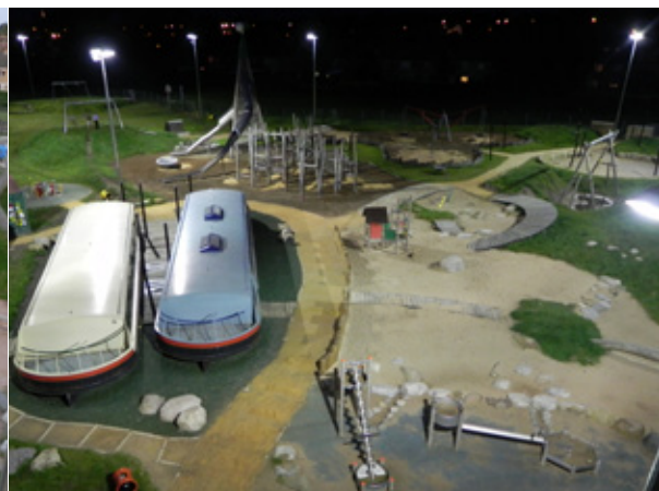
Even when housing is quite close to a floodlighting installation, with careful design and accurate aiming of the luminaires, nuisance through light spill and glare can be minimised
