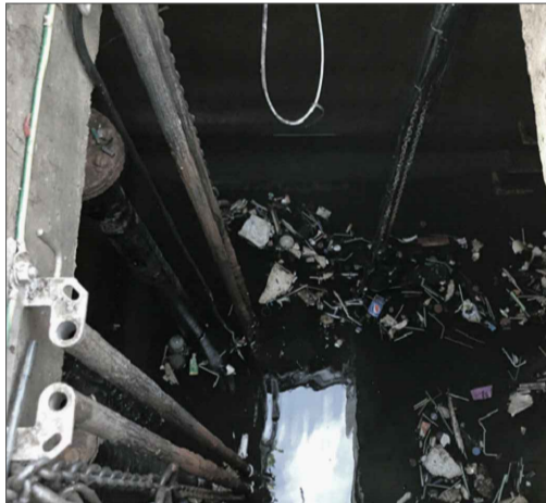
9. SURFACE WATER SEWER (CIRCA 2000M Ø)
