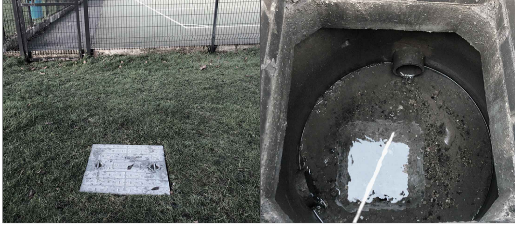
2. SURFACE WATER MANHOLE MH02
