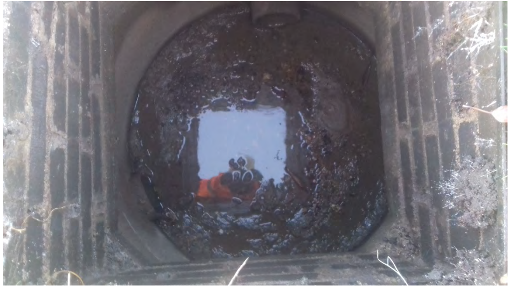
Photograph 7.6 Inside manhole chamber located to south west of pitch
