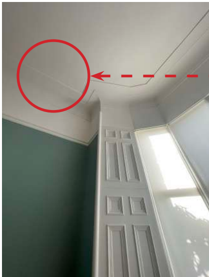
Living room existing cornice
