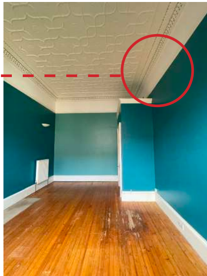
Bedroom 3 existing cornice
