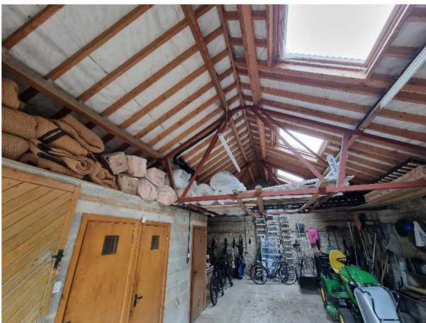
Photograph 5. The internal space of the outbuilding.
