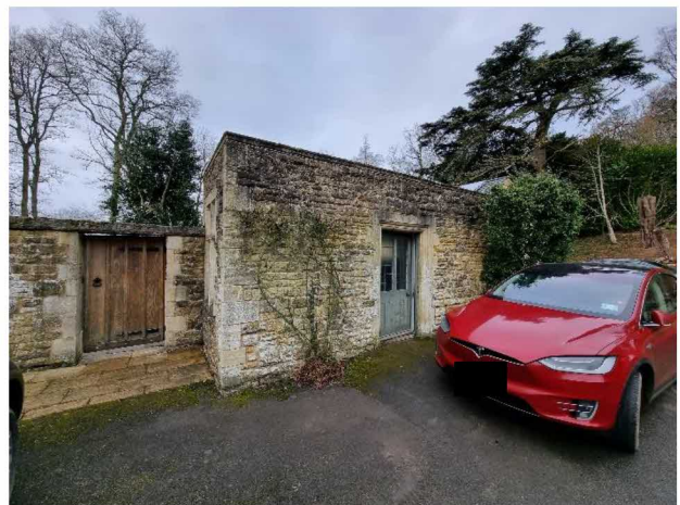
Photograph 6. The pool building viewed from the east.
