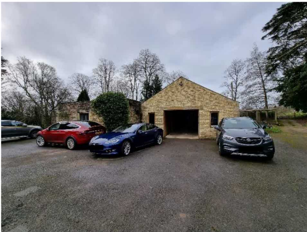
Photograph 3. The outbuilding, and area of hard-standing, viewed from the east.
