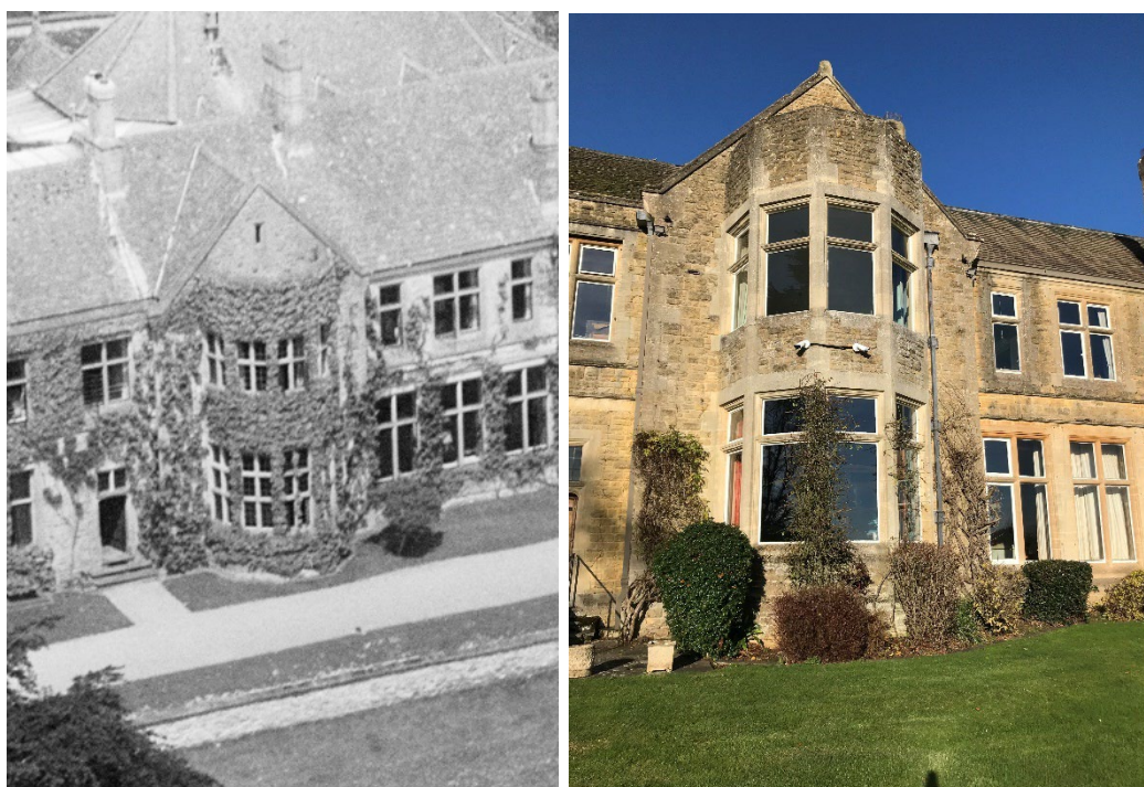
Figure 7: Lutyens bow window in 1951 (left, HE Archive ref: haw_9419_10) and today. The upper windows have had their sills lowered and central mullion removed, the lower windows have a central mullion and lower transom removed. All are currently double glazed.
