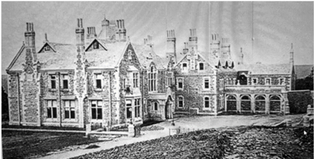
Figure 4: 1872 photograph of the entrance front (Historic England OP11030) Note no doorway in the eastern façade where the location of the present doorway is circled.
