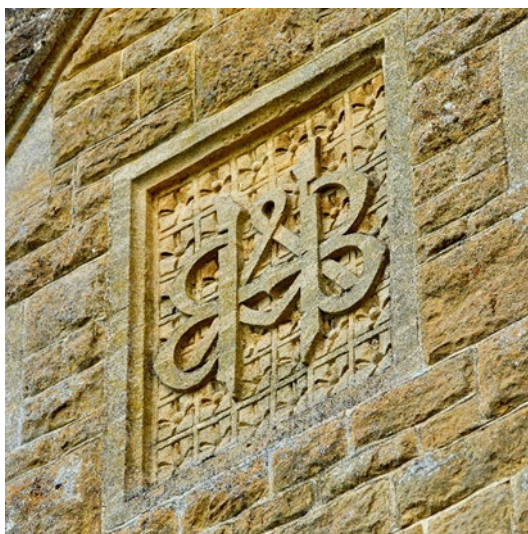
Figure 8: H A Brassey's initials on the eastern facade
