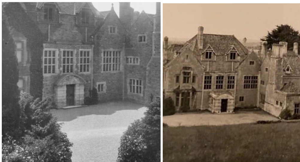
Figure 6: Comparative photographs of the porch showing (left) Lutyens' relatively shallow depth, and (right) photo of c. 1970 showing extended form with side window just visible.
