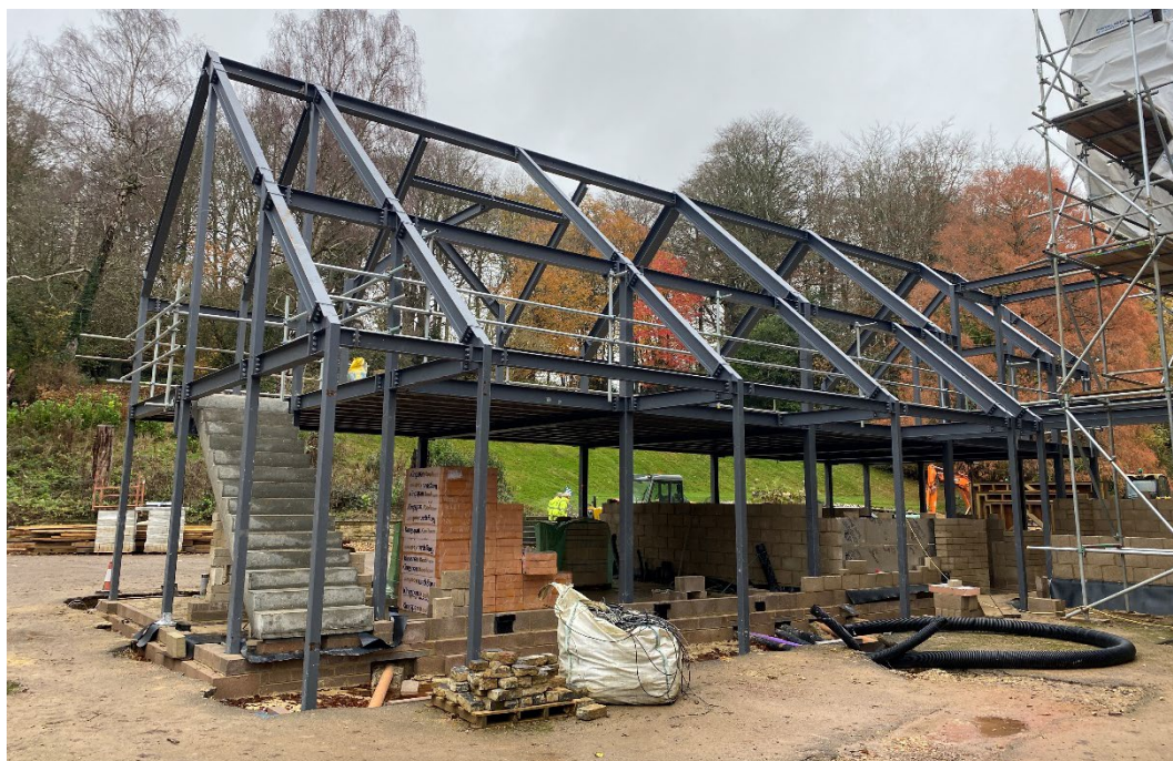
Figure 3: Construction of the framework for consented annex extension, January 2024.
