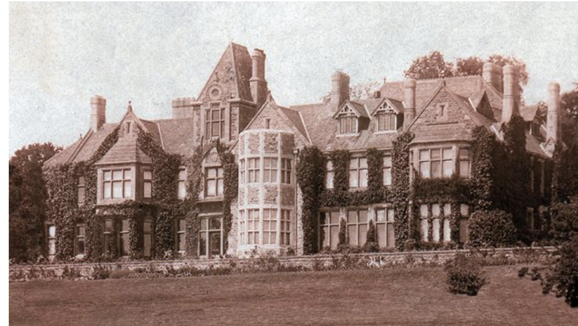
Images from the Henry Taunt Collection held in the Oxfordshire Picture Collection showing Cope Hill House after Lutyens' work.
