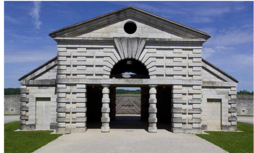
Gatehouse of the Saline Royale, Arc-et-Senans, Claude-Nicolas Ledoux Ledoux gatehouse, with its rusticated bands and segmented head and recessed masonry panels.
