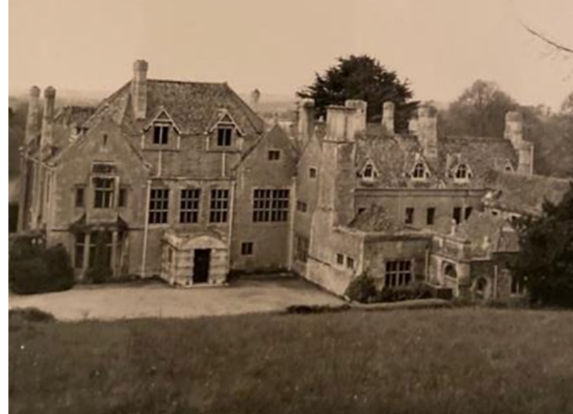
Photo of early 1970s, with service wing still in existence. Note the length of the porch is clear, more closely resembling the original 1871 porch length (photo credited from HCUK Group Heritage Statement, Feb 2022, page 15)
