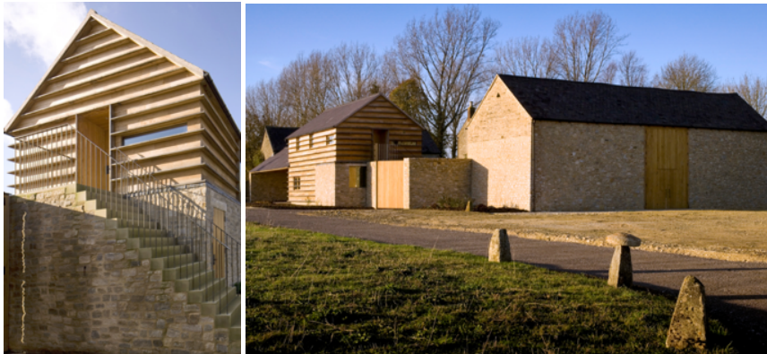
Above images show modern use of banding at GII listed farmhouse in the Cotswolds, by James Gorst Architects.
