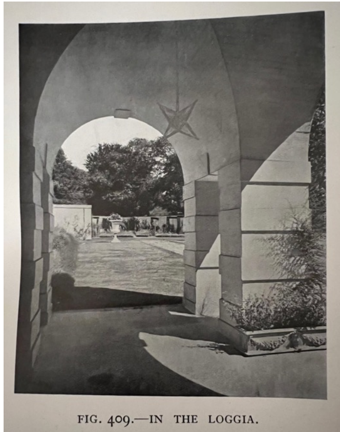
Image above showing example of Lutyens' rusticated bands and series of archways, at Nashdom.
