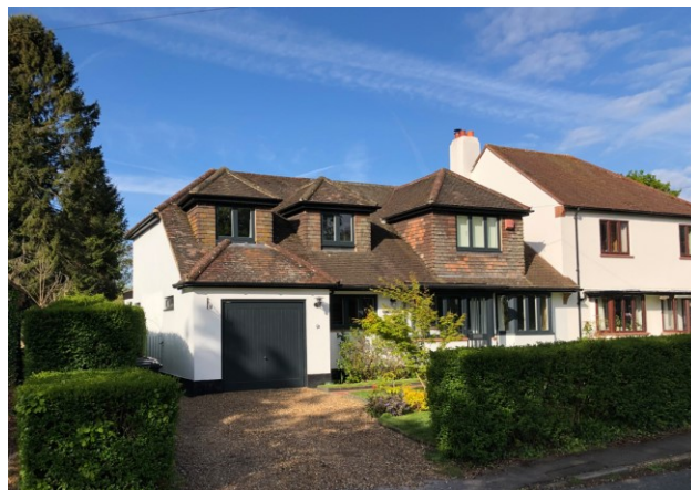
Existing pair of cottages
