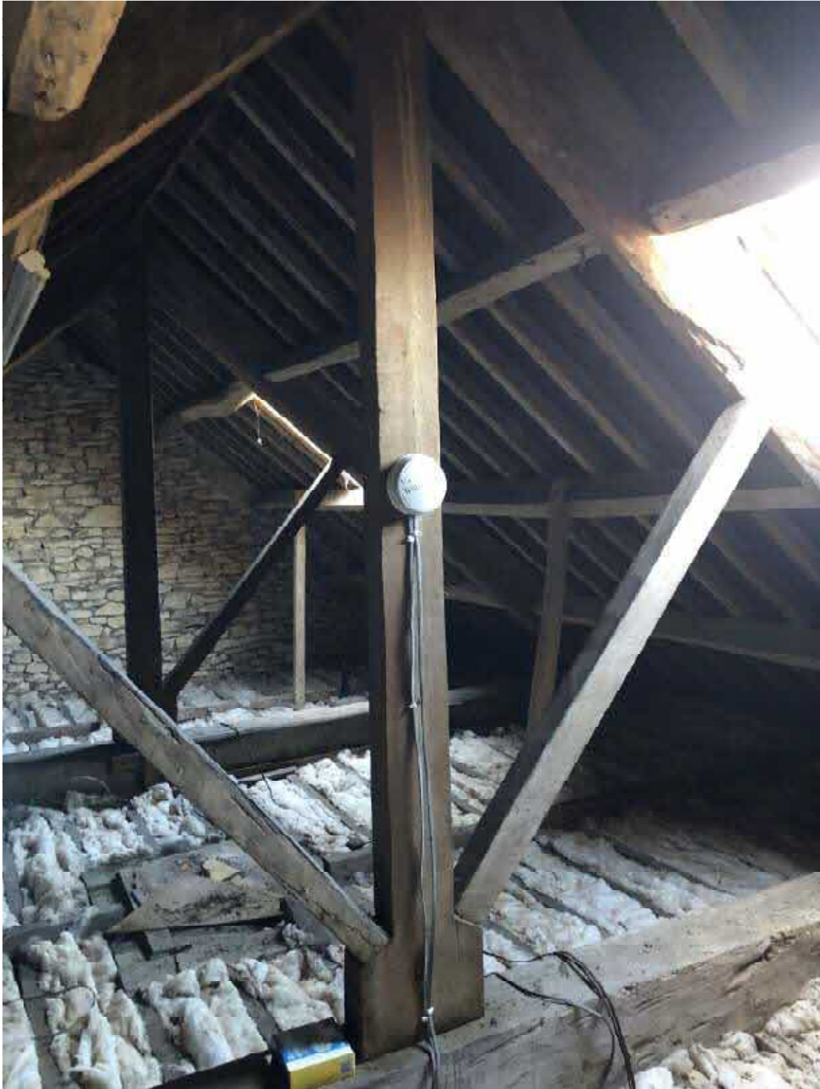
Fig 12: King post truss in the roof space.
