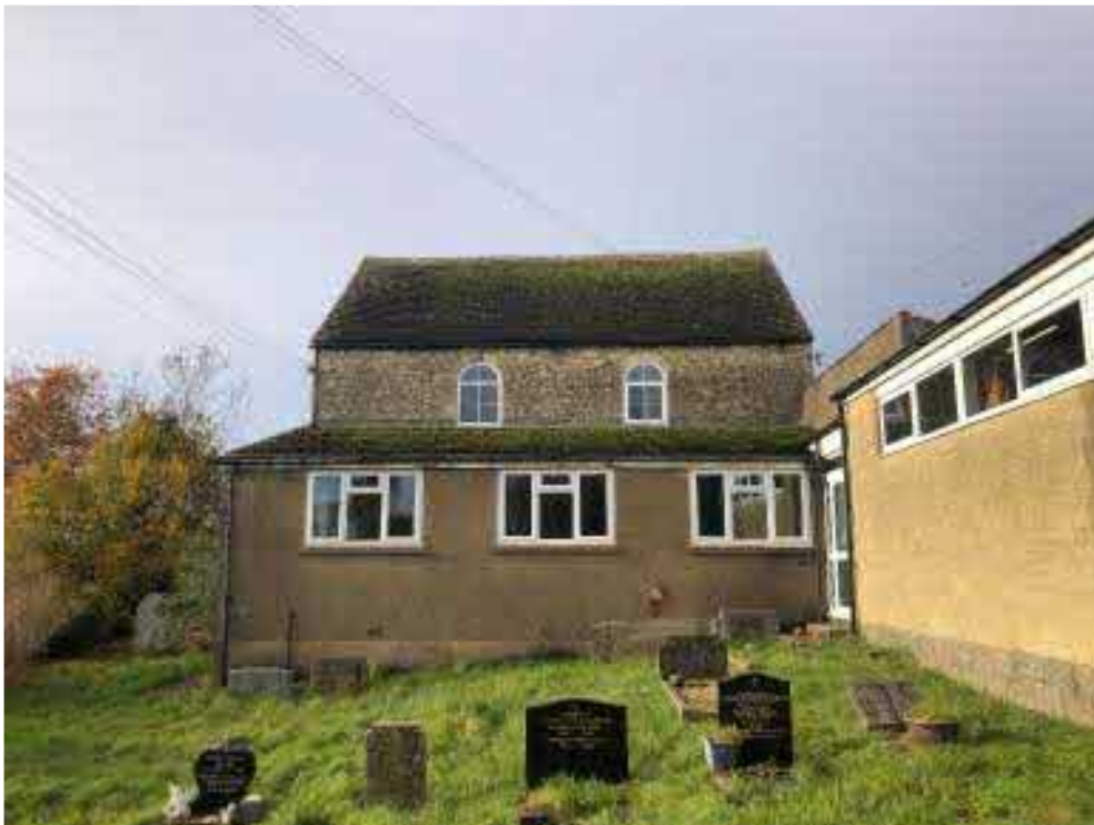
Fig 6: View of east side of the church showing the lean-to extension.
