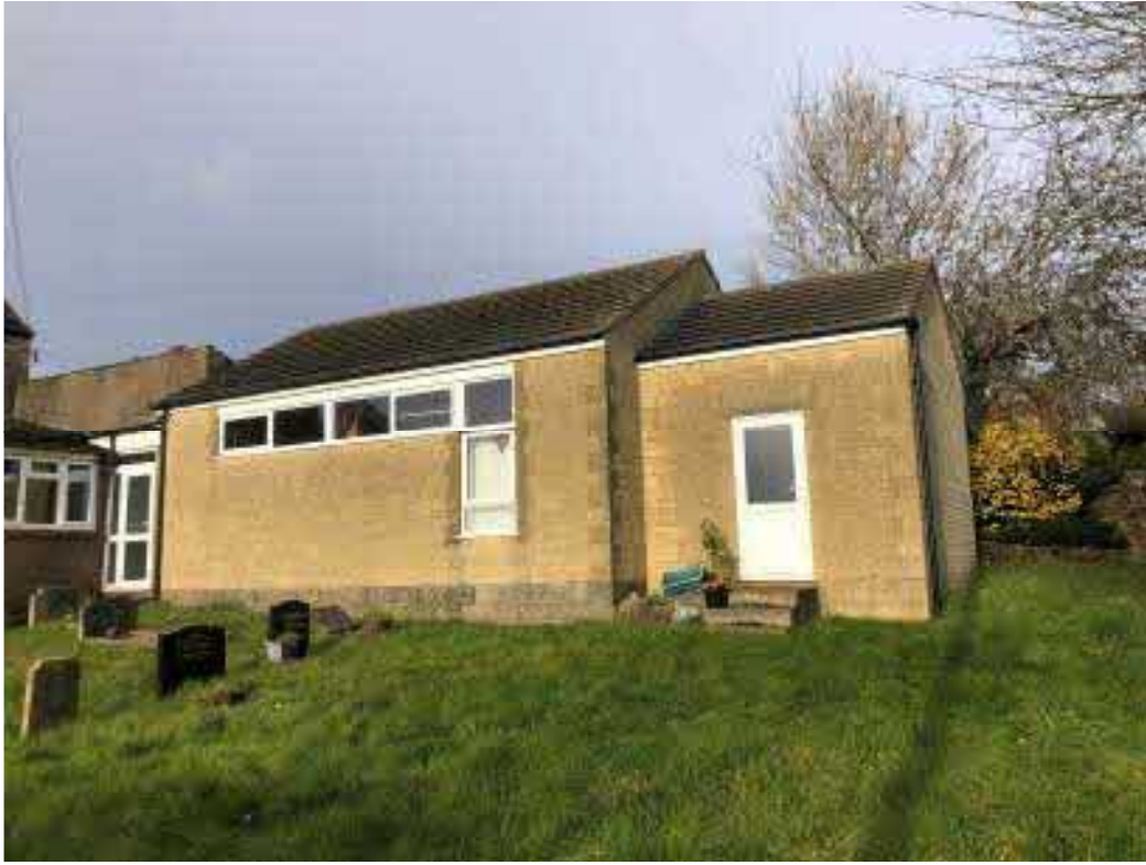
Fig 7: View of the back of James Gibbs Hall.
