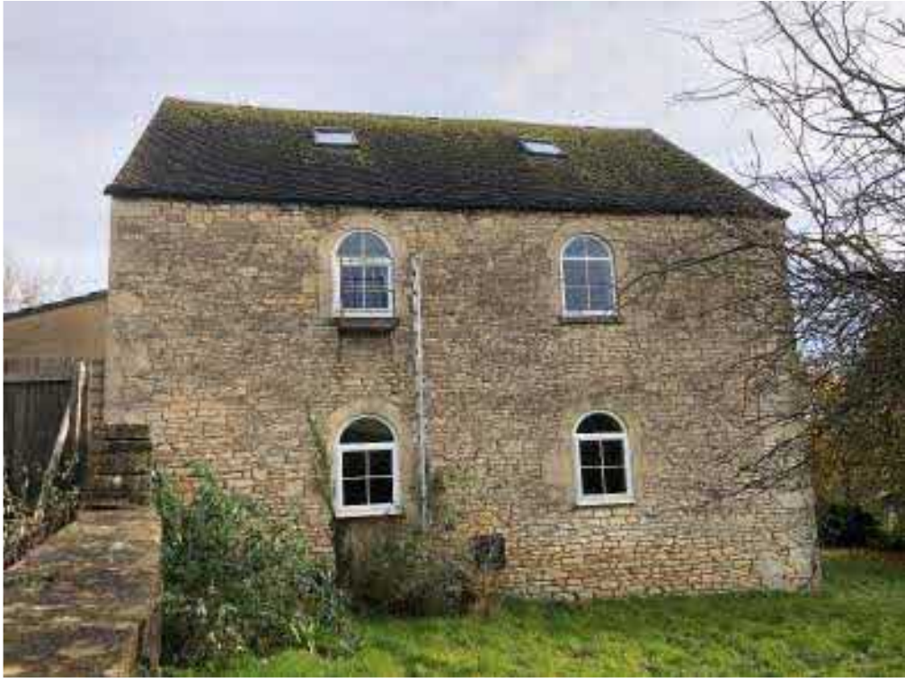
Fig 9: West facing wall of the church.
