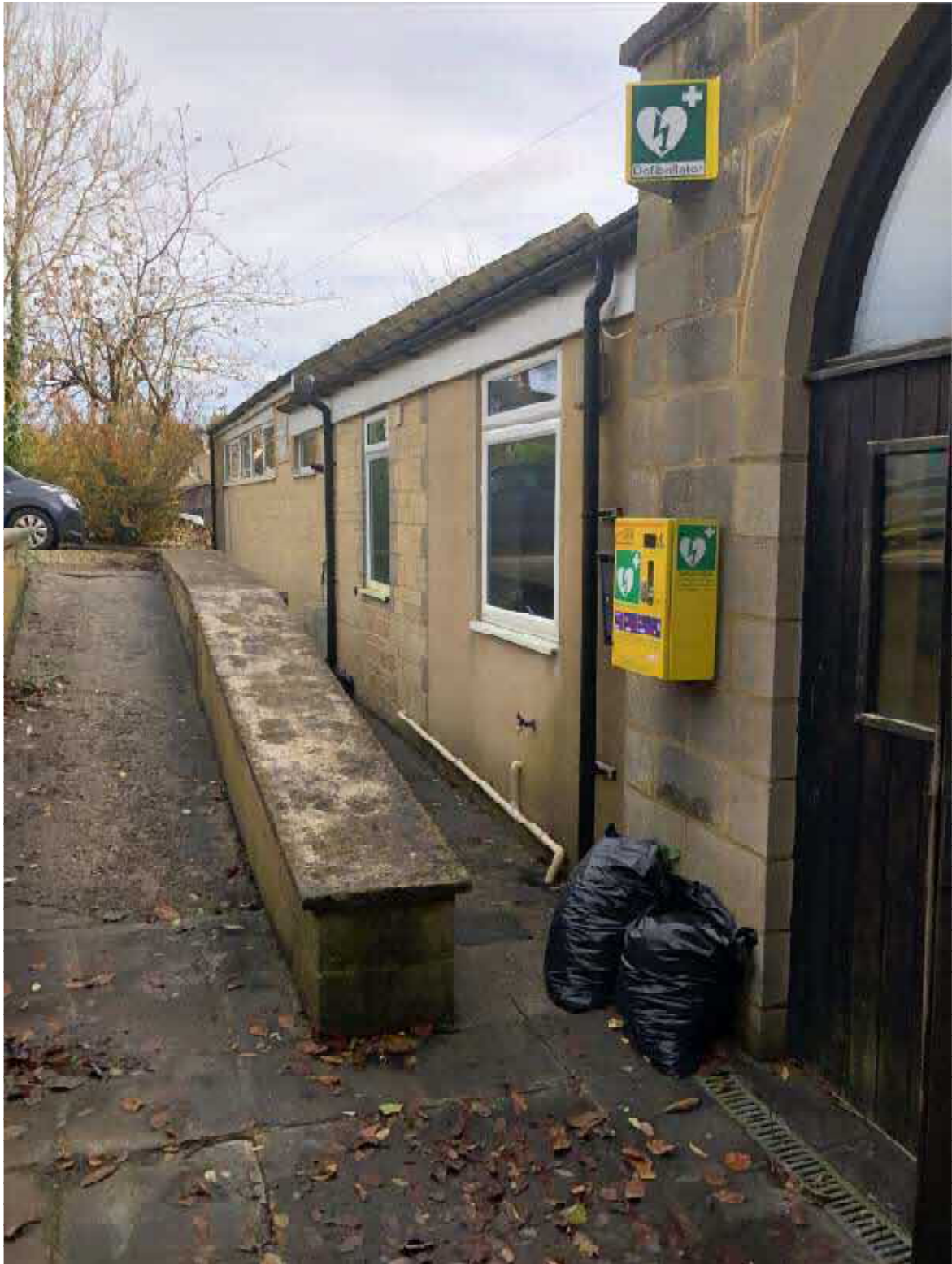
Fig 11: View along the front of the buildings.
