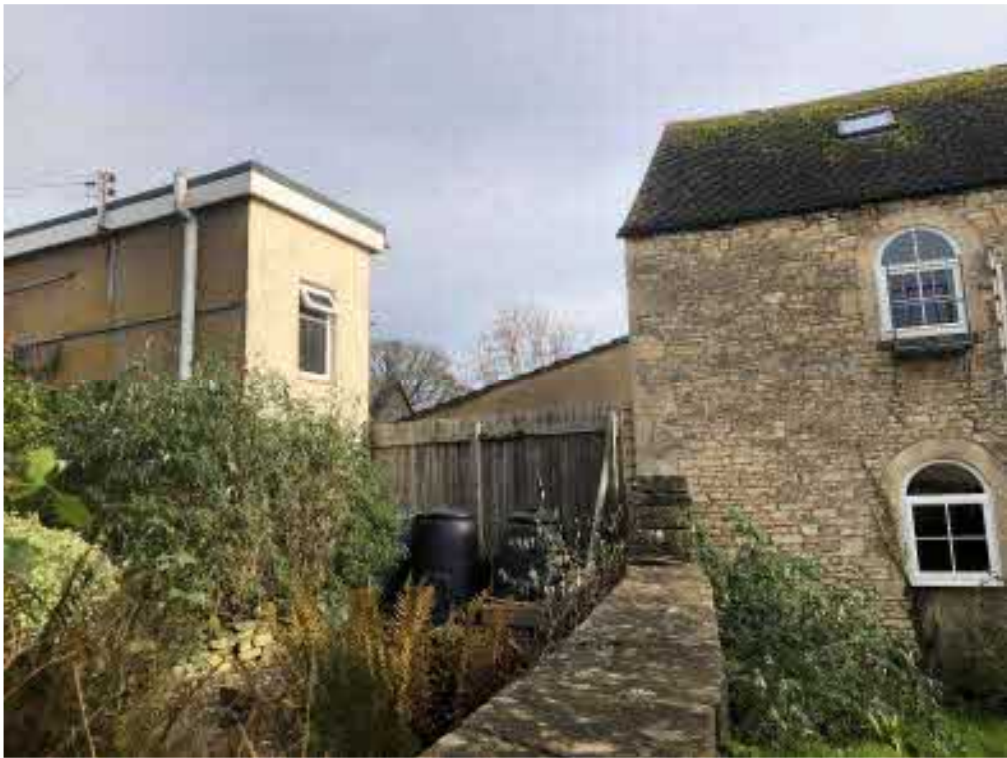
Fig 10: View from the west showing the church and their neighbouring property.
