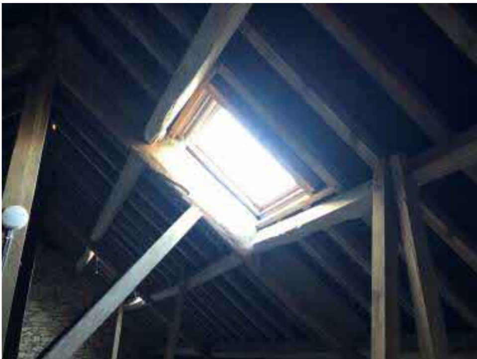
Fig 14: Existing rooflight in roof space.
