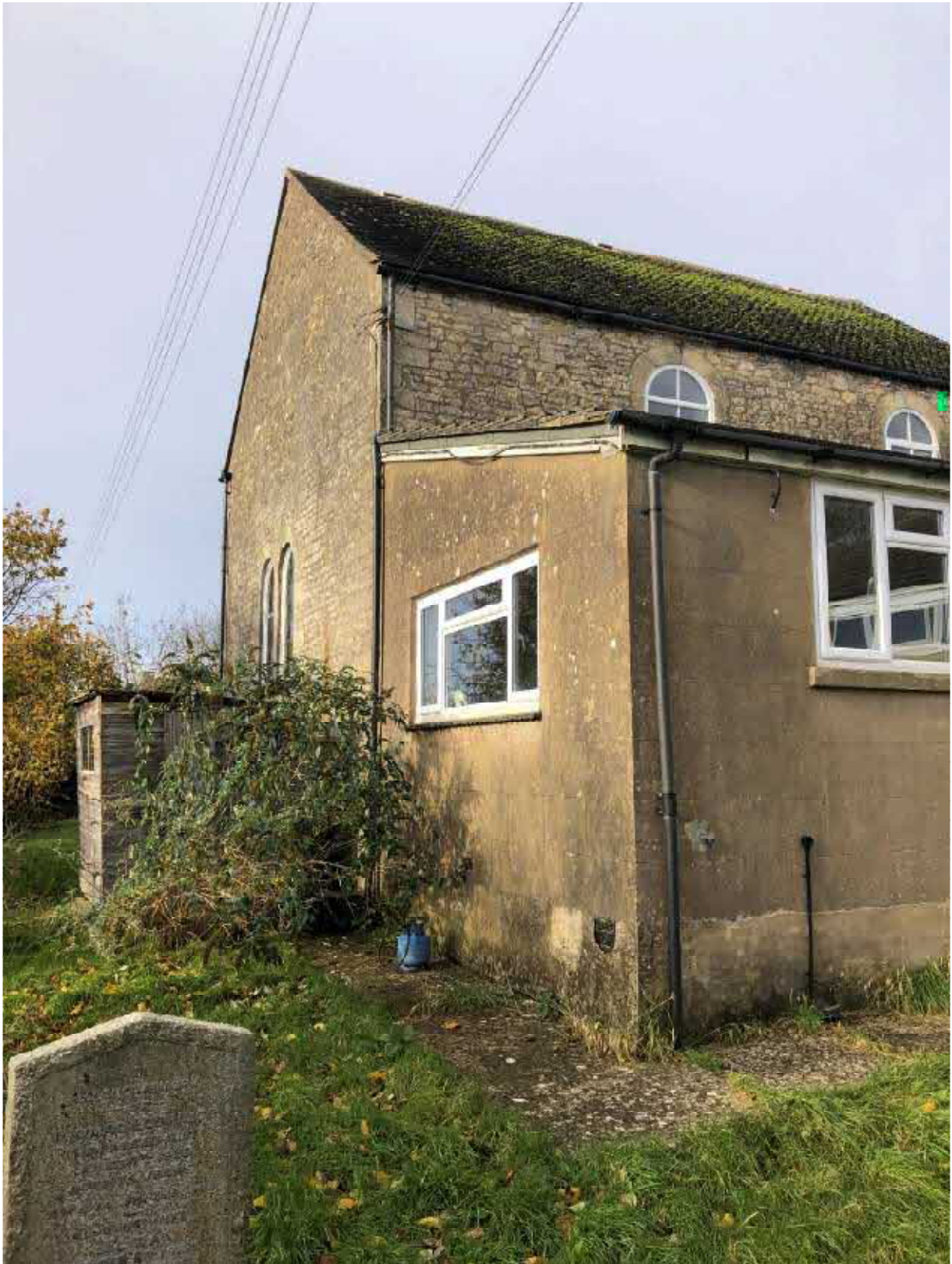
Fig 8: View of south wall of church and the lean-to extension.
