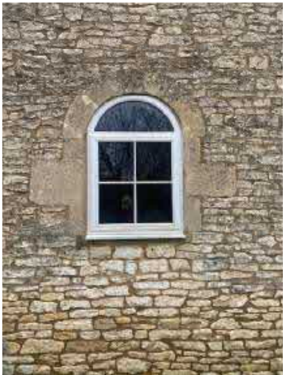
Fig 16: Typical replacement window in the church building.
