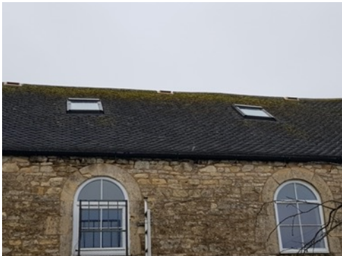
Photo 5: Proposed site of new skylights - West facing roof aspect
