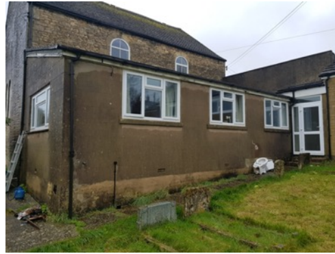
Photo 2: Mono-pitched extension located at the eastern elevation
