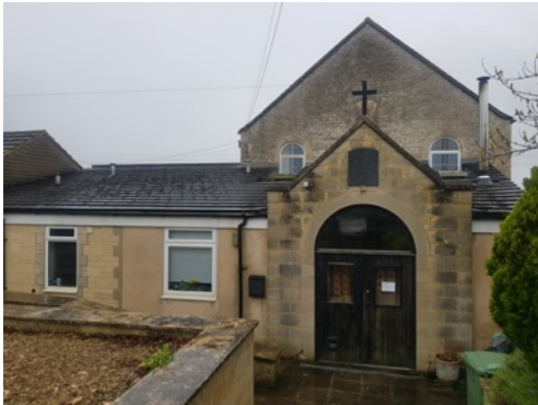
Photo 1: Main entrance at north facing elevation
