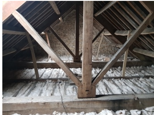
Photo 8: Internal view of loft space
