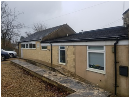
Photo 3: Northern elevation of single storey extension
