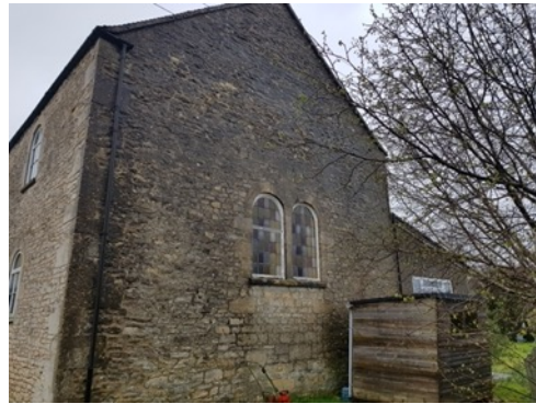
Photo 4: Proposed site of new window - South facing gable end
