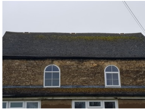
Photo 6: Proposed site of new skylights - East facing roof aspect
