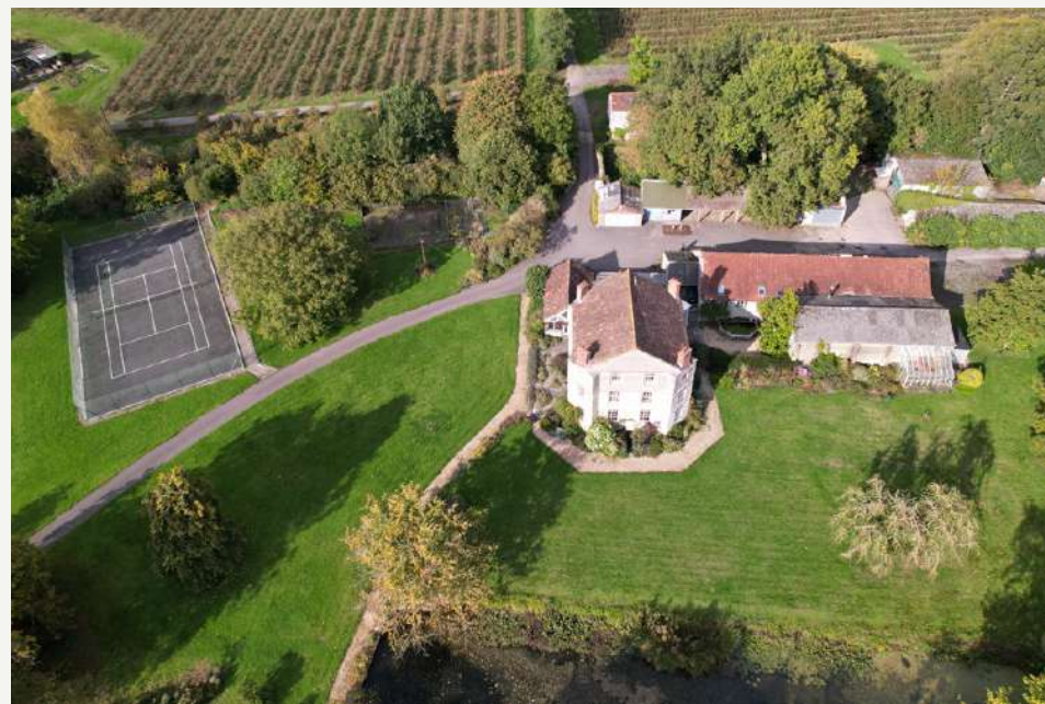
VIEW FROM THE SOUTH
