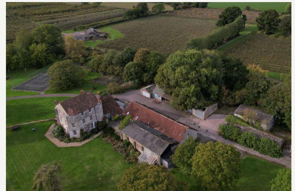
VIEW FROM THE SOUTH EAST
