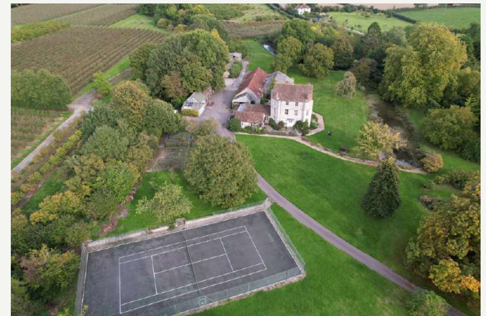
VIEW FROM THE WEST
