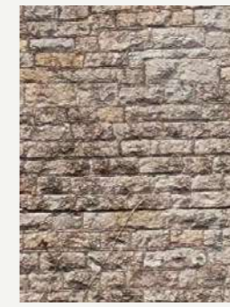
EXISTING LIAS STONE- WORK
