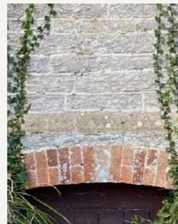
EXISTING RED BRICK INTERVENTIONS RE- POINTED
