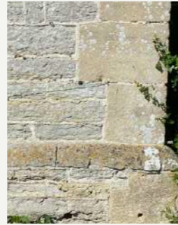
EXISTING LIAS STONE CAREFULLY RE POINTED
