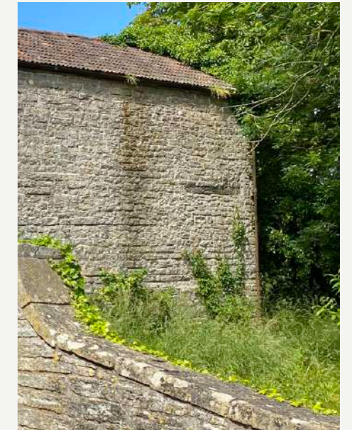
SOUTH ELEVATION WITH A LINTEL OVER AN EXTANT DOORWAY
