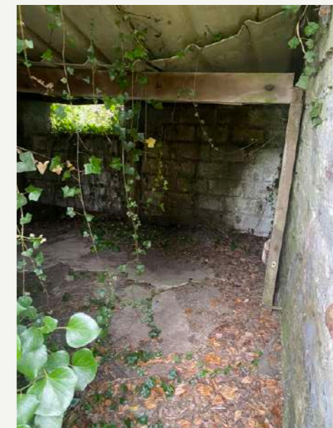
A MODERN LEAN-TO ADDITION TO THE WEST.
