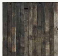
TIMBER POSTS AND INFILLS
