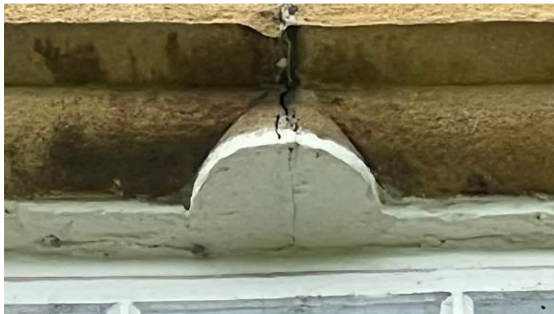
Figure 10 Detail of south-west, second-floor window mullion profile.
