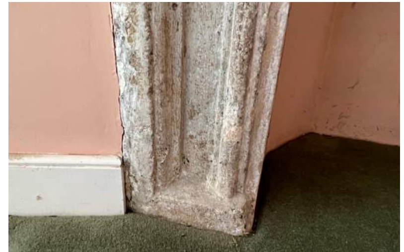
Figure 90 Detail of fireplace in north-west ordinal projection.
