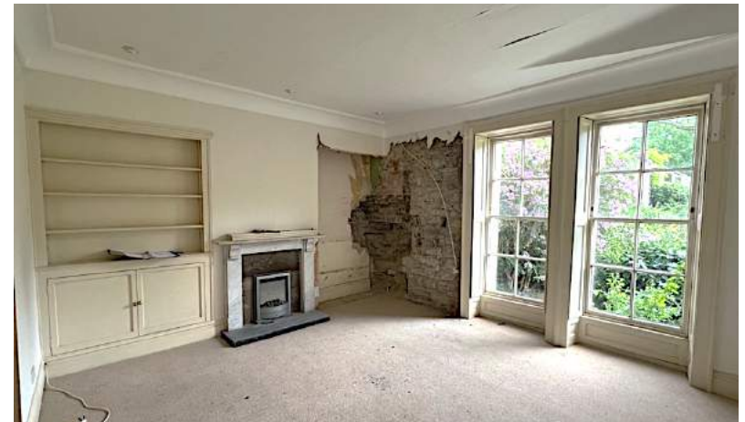
Figure 70 Dining room, facing north-east.
