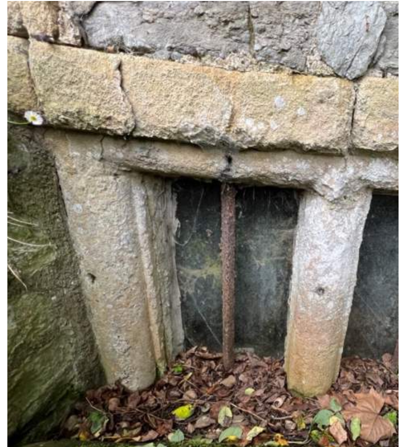
Figure 11 West front, detail of cellar window.
