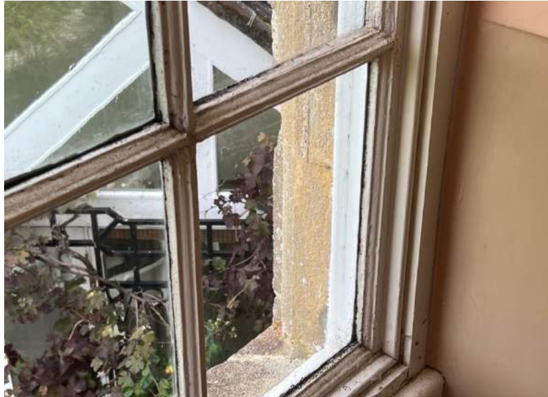
Figure 12 Detail of north-west, first-floor window.
