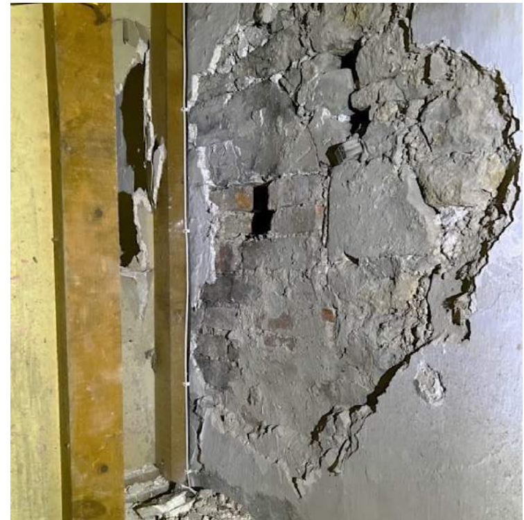
Figure 61 Remains of fireplace behind 19 th -century stair.
