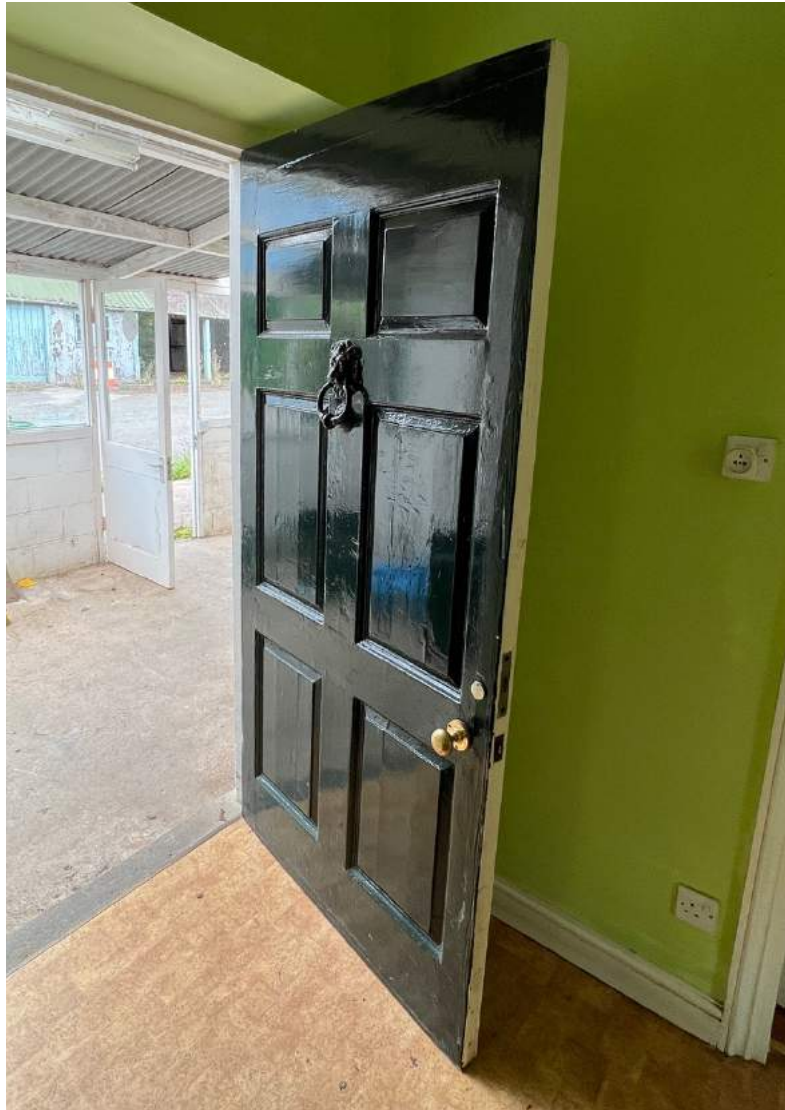
Figure 107 Reused 18th-century external door.
