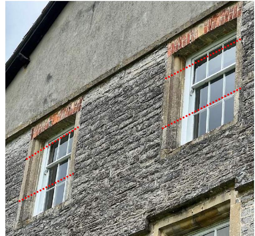
Figure 26 South elevation, second-floor windows; consistent lower & upper breaks marked.
