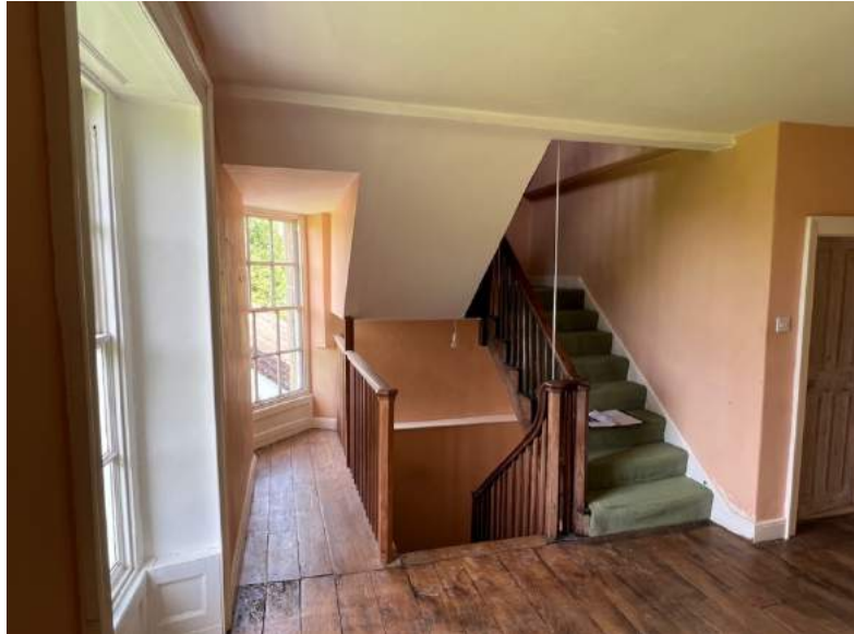
Figure 79 Stair from first-floor landing.
