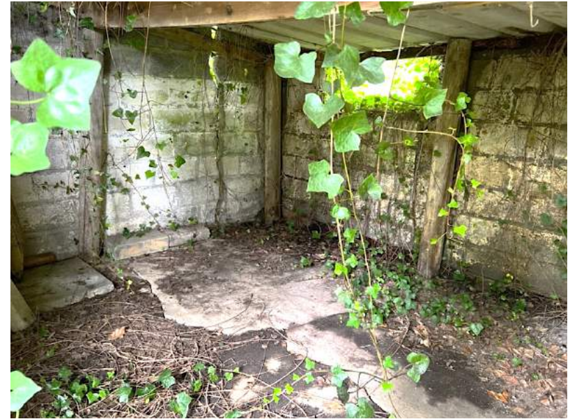
Figure 122 Little Stone Barn, eastern addition.
