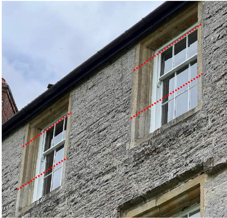
Figure 27 West elevation, second-floor windows; consistent lower & upper breaks marked.
