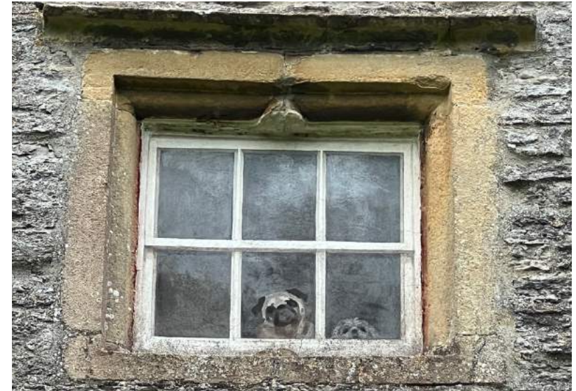
Figure 22 Second floor, south-east blind window.
