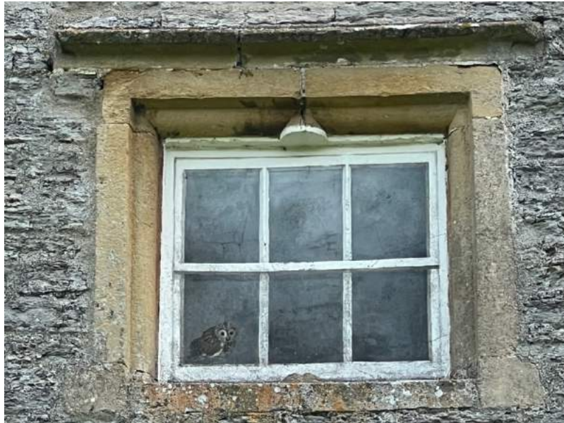
Figure 9 South-west, second floor window.
