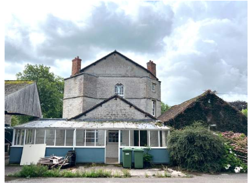
Figure IO4 North wing, north elevation.
