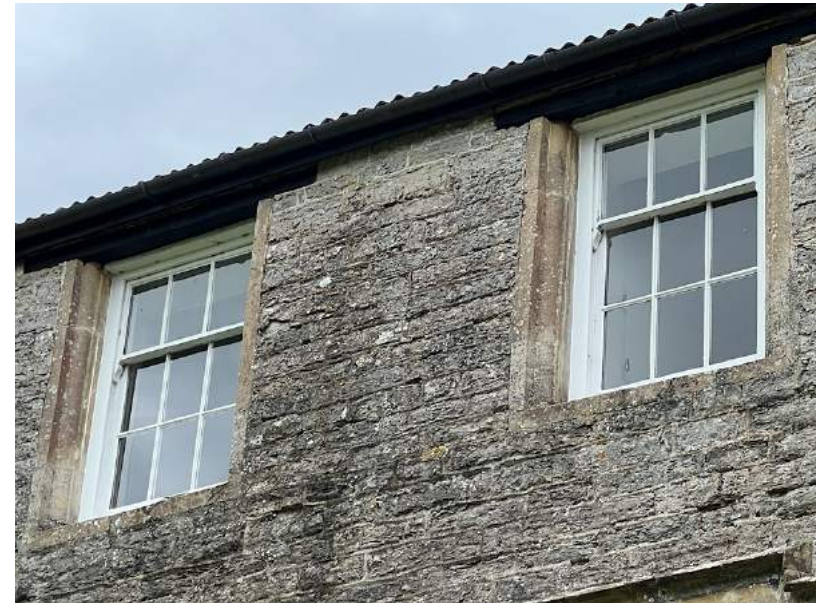
Figure 24 East elevation, second-floor windows.
