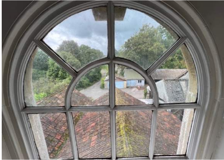
Figure 94 Detail of upper sash of the former stair window.
