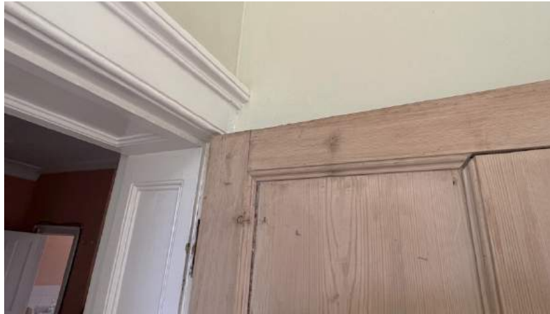
Figure 66 19th-century door (dipped) & lining.
