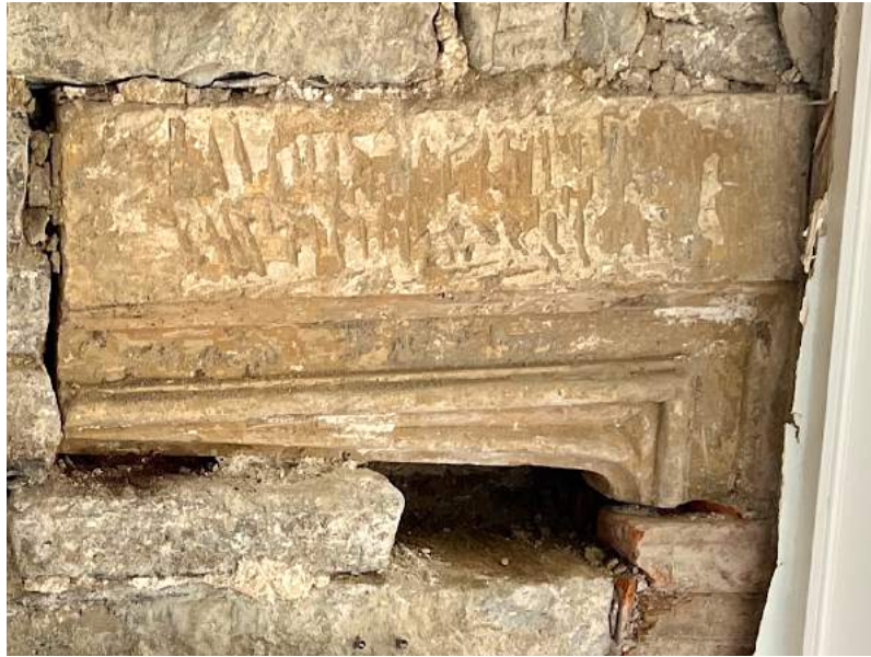
Figure 84 Detail of head of fireplace in north-east room.
