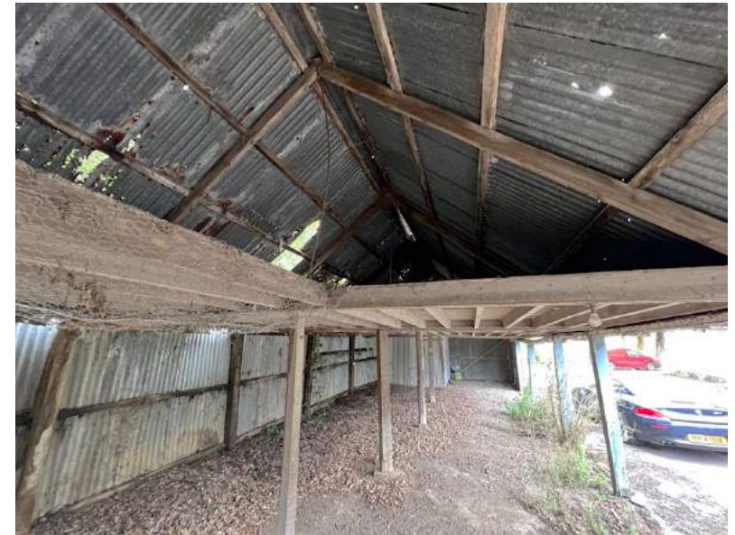
Figure 131 Cart /hed, interior facing east.
