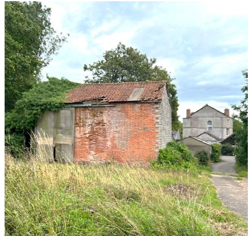
Figure 120 Little Stone Barn, from the north.
