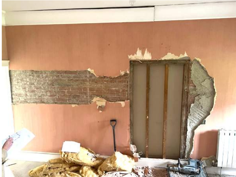
Figure 57 Hall, south wall, showing brick construction & blocked door to south-west room.
