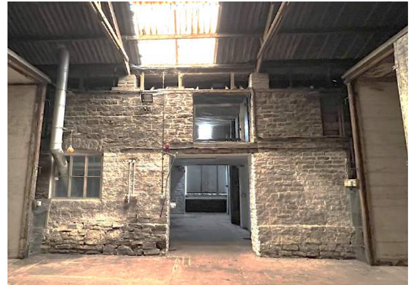
Figure 129 Original south elevation of Apple Barn, now within Concrete Barn.
