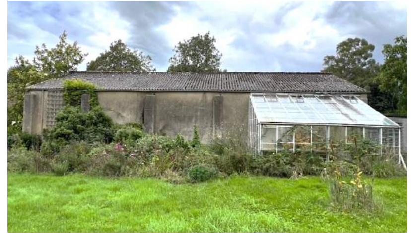
Figure 128 Concrete Barn, south elevation.
