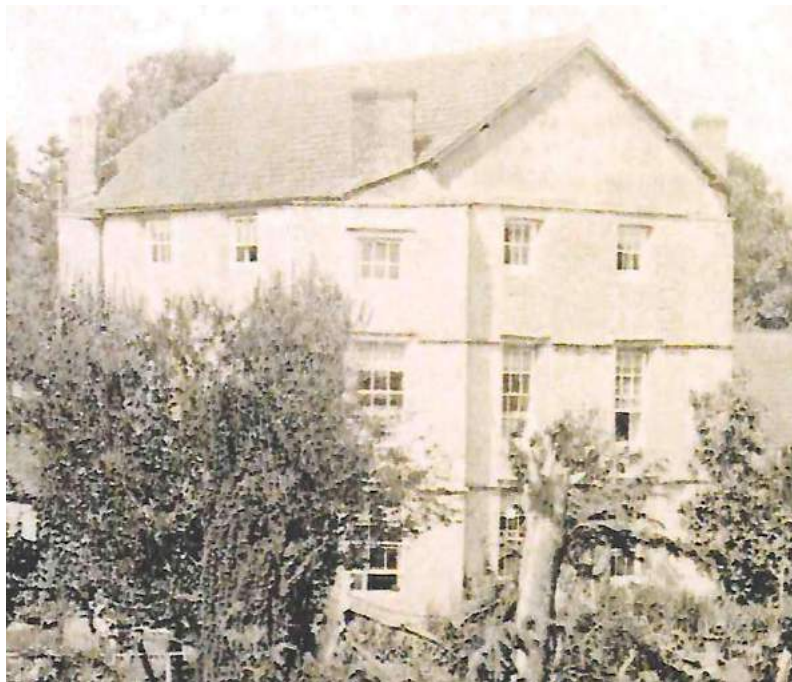
Figure 25 Undated, possibly early-20 th century photograph (the ordinal blind window has now been painted), showing higher sills on the second-floor windows on the west & south elevations.
