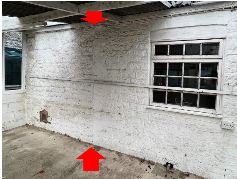
Figure 105 North elevation, showing straight joint & quoins.
