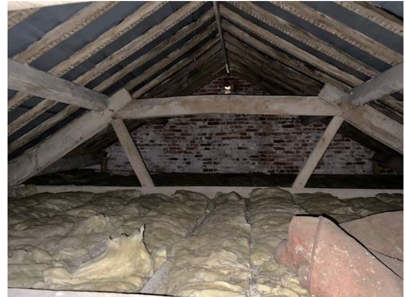
Figure 98 Within the roof, facing south.
