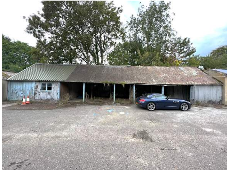
Figure 130 Cart /hed, south front.
