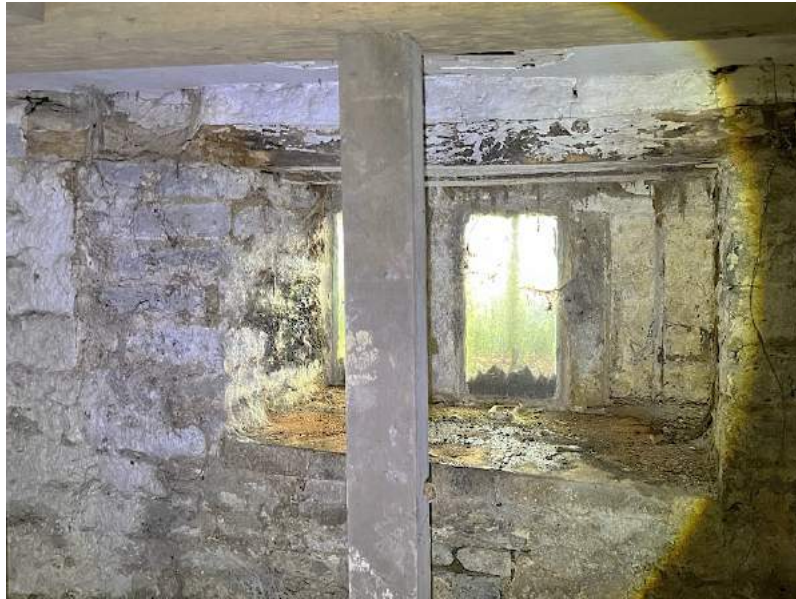
Figure 51 South-west window, with northern light blocked, & splay infilled.
