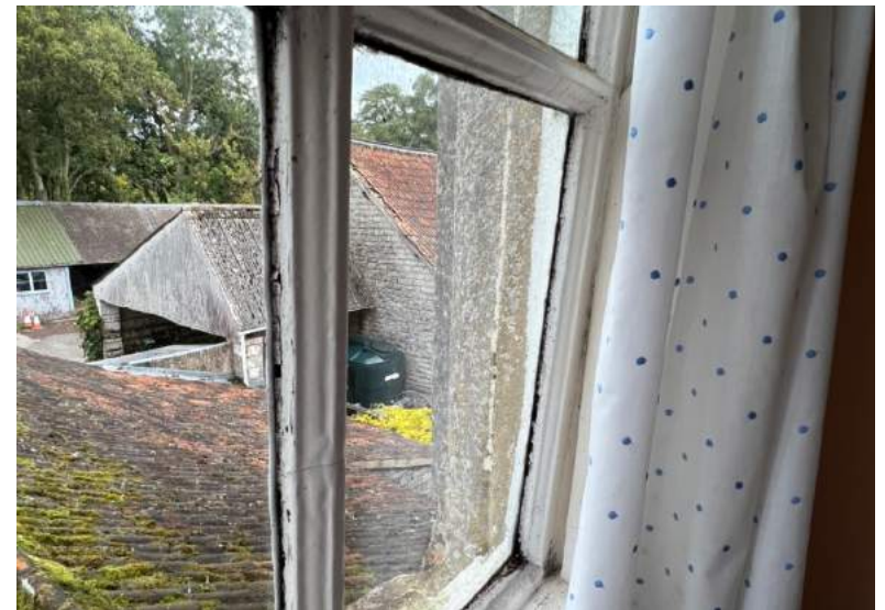
Figure 81 Detail of stair window.
