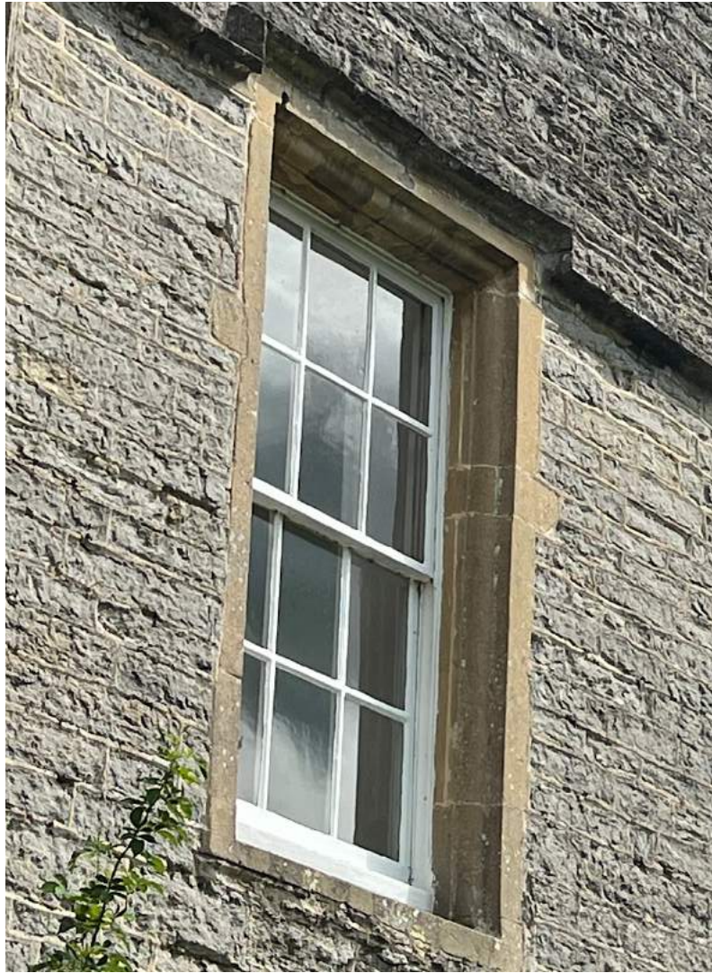
Figure 8 South front, first-floor window.
