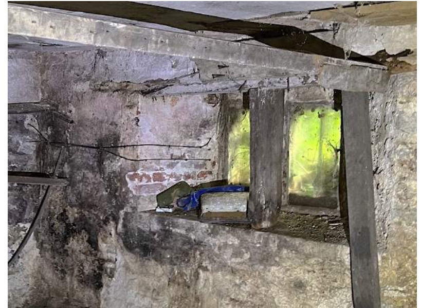
Figure 52 East window, with red brick infill to north (left).
