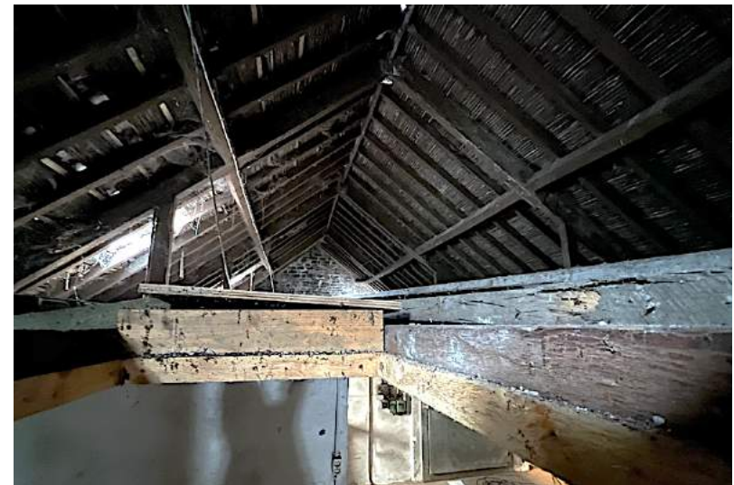
Figure I26 Apple Barn, roof structure in western half, facing east.
