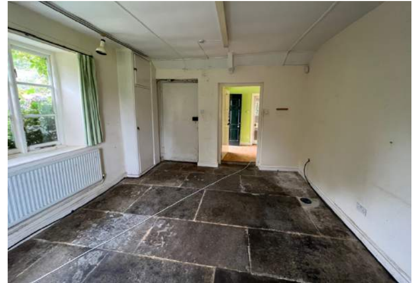
Figure I11 North-east room facing east, with retained stone floor.
