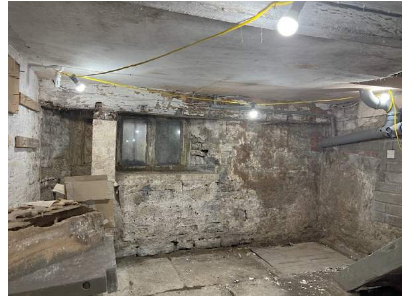
Figure 47 North-west room, west wall with reused beam.
