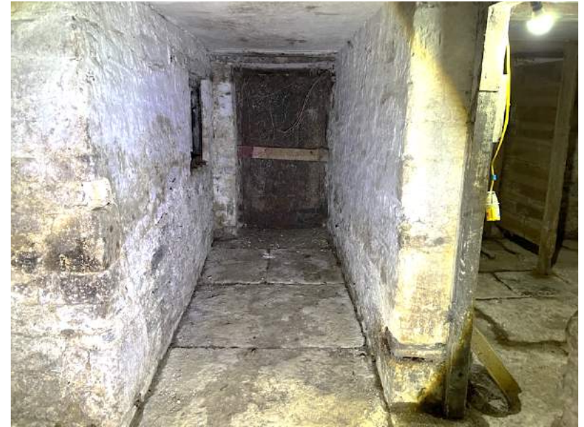
Figure 54 passage facing south to external cellar door.
