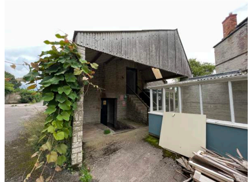
Figure 165 Existing Conservatory & link to Apple Barn.
