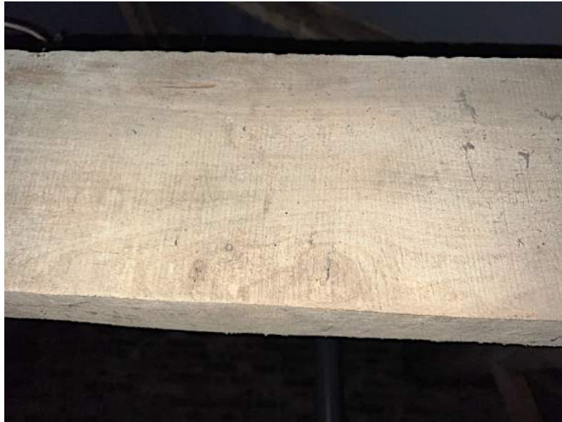
Figure 99 Detail of collar, with characteristic markings for a timber that was pit-sawn.
