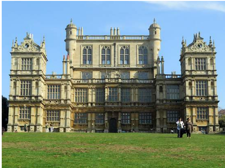
Figure 147 Central prospect room raised above the hall clerestory, Wollaton Hall, Nottinghamshire; Robert Smythson, 1580-.
