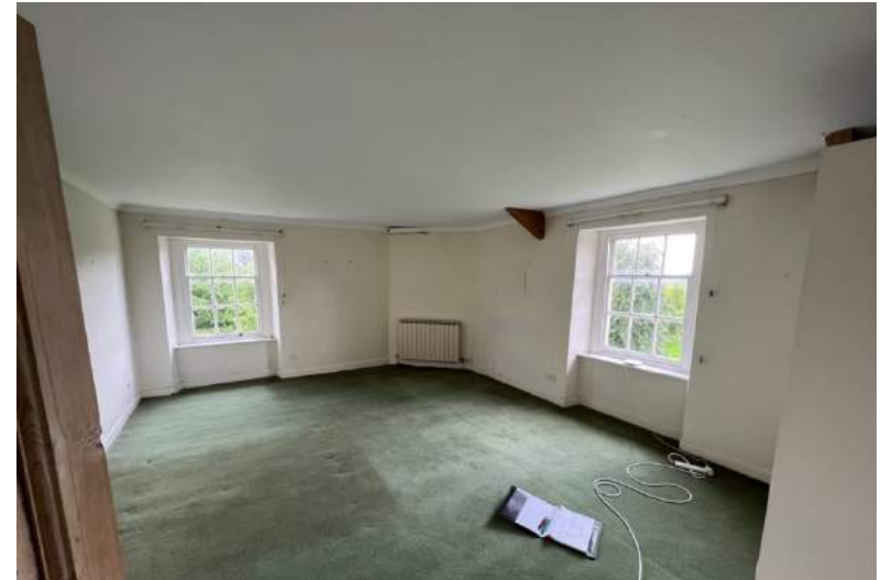
Figure 95 South-west room (with modern lowered ceiling).
