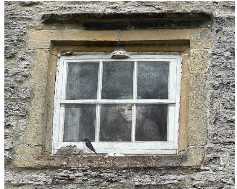
Figure 20 Second floor, north-west blind window.
