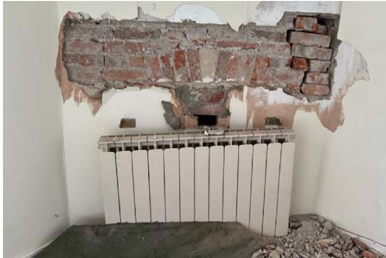
Figure 91 19 th -century fireplace in the south-west projection.
