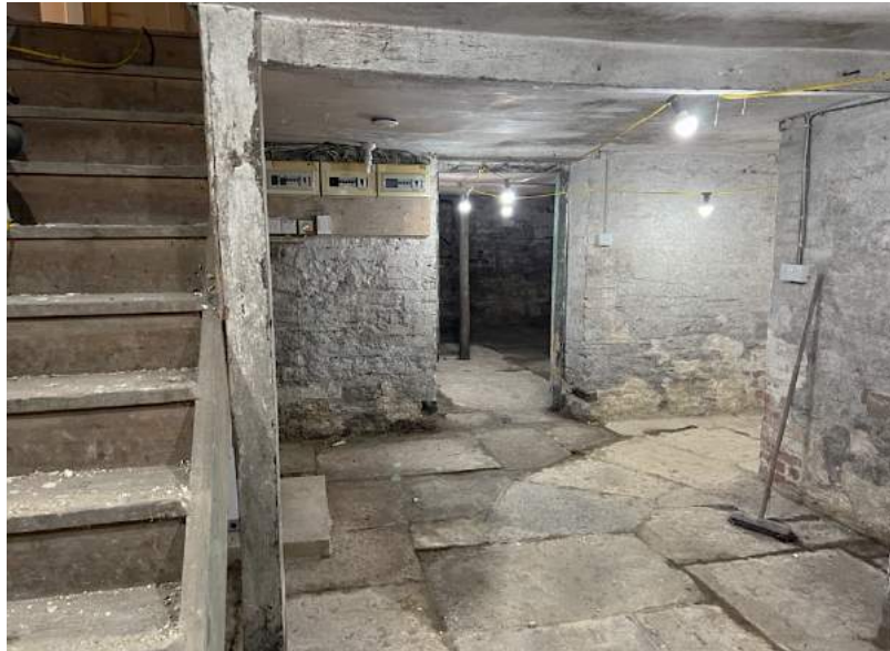
Figure 46 Cellar, north-west room, facing east.
