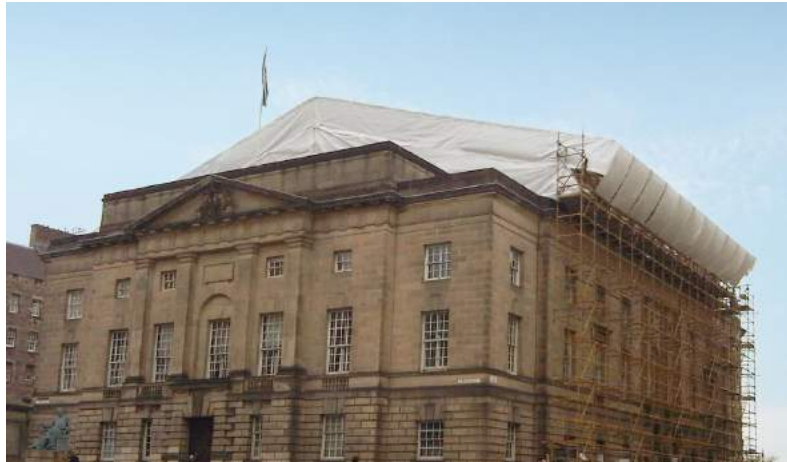
Figure 139 Temporary roof (High Court of Justiciary, Edinburgh).
