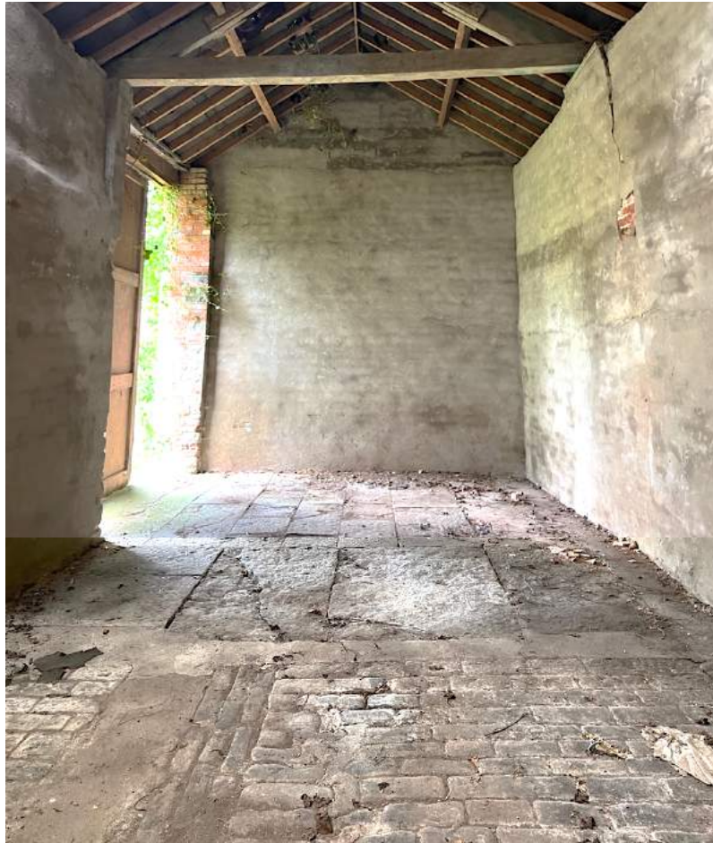
Figure 121 Little Stone Barn, interior facing east.
