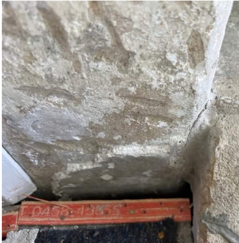
Figure 86 Detail of left jamb of the south-west fireplace, showing the fine coat of plaster that extends down below the present floor level.
