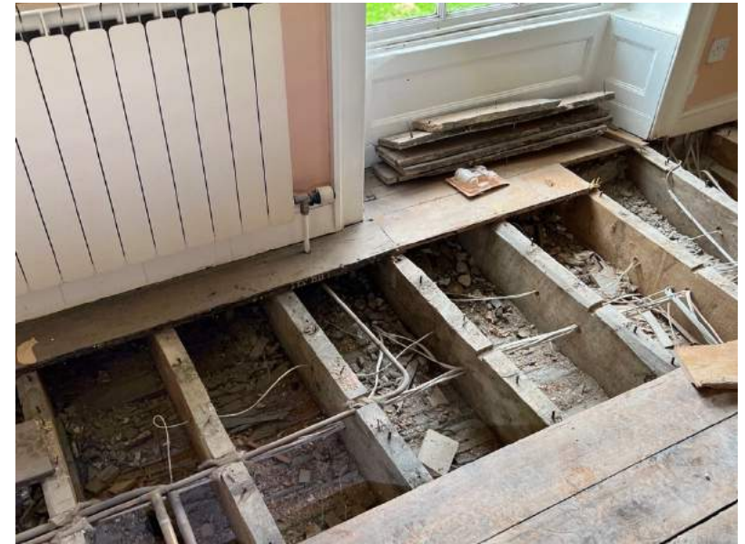
Figure 50 Floor structure above south-east room, from drawing room.
