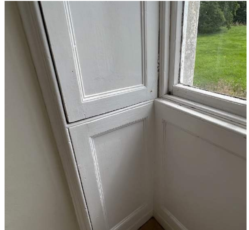
Figure 65 19 th -century window lining, 20 th -century sash window.
