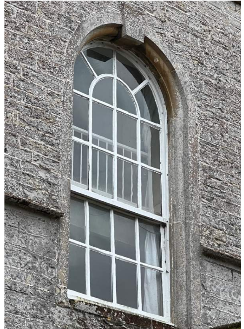
Figure 19 North front, stair window, showing glazing slot on the reveal.
