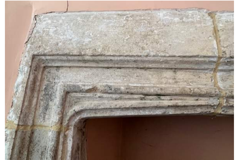
Figure 89 Detail of fireplace in north-west ordinal projection.
