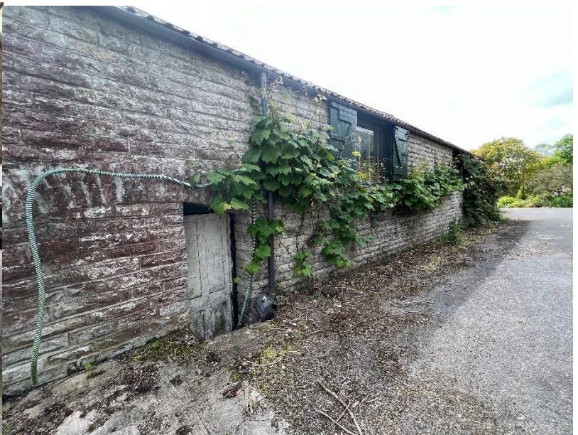
Figure 6: External view of the Apple Barn
