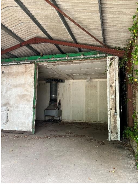
Figure 10: Steel portal frame shed
