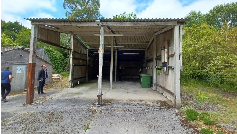
Figure 9: Precast Concrete Shed
