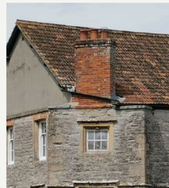
AWKWARD CHIMNEY AND GUTTER JUNCTIONS ARE UNSIGHTLY AND HAVE RESULTED IN WATER INGRESS DAMAGING HISTORIC FABRIC.
