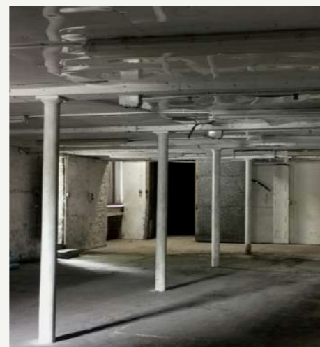
APPLE BARN - GROUND FLOOR WITH STEEL COLUMNS SUPPORTING THE FIRST.
