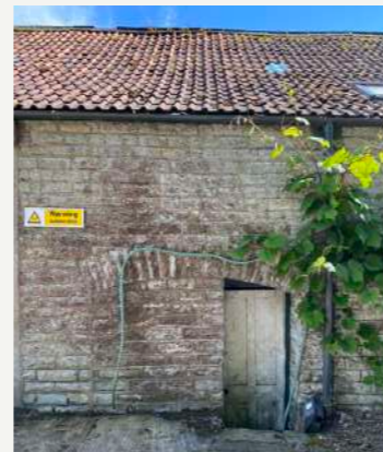
D EXISTING STONE ARCHED OPENING TO BE OPENED UP WITH NEW FIXED GLAZING. THE STEPS ARE CONTEMPORARY WITH THE NEWER DOOR.
