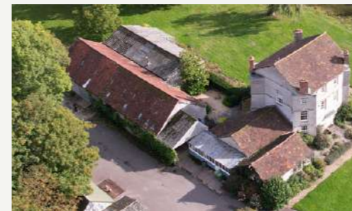
AERIAL VIEW OF ALL THE EXTENSIONS TO THE NORTH OF THE MAIN HOUSE
