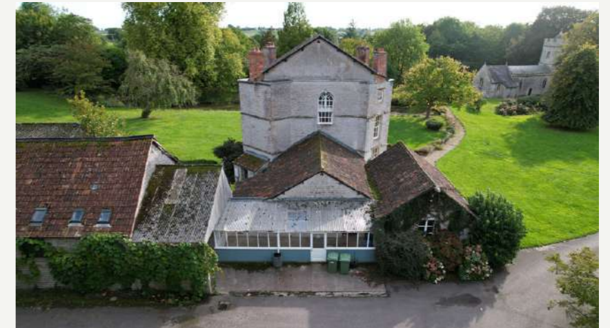
AERIAL VIEW OF EXISTING COLLECTION OF EXTENSIONS AND LEAN-TO'S
