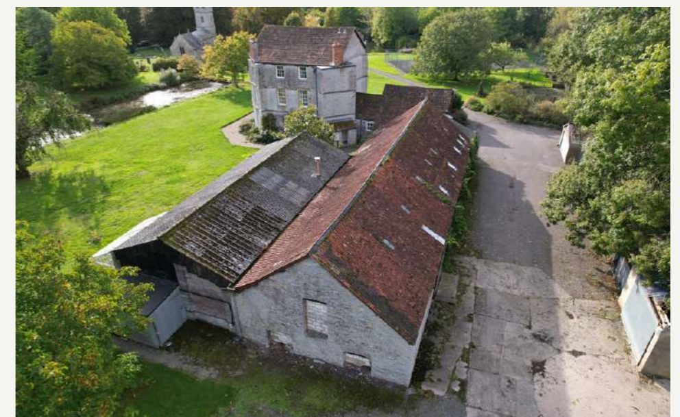
ARIEL VIEWS OF THE APPLE BARN AND CONCRETE BARN
