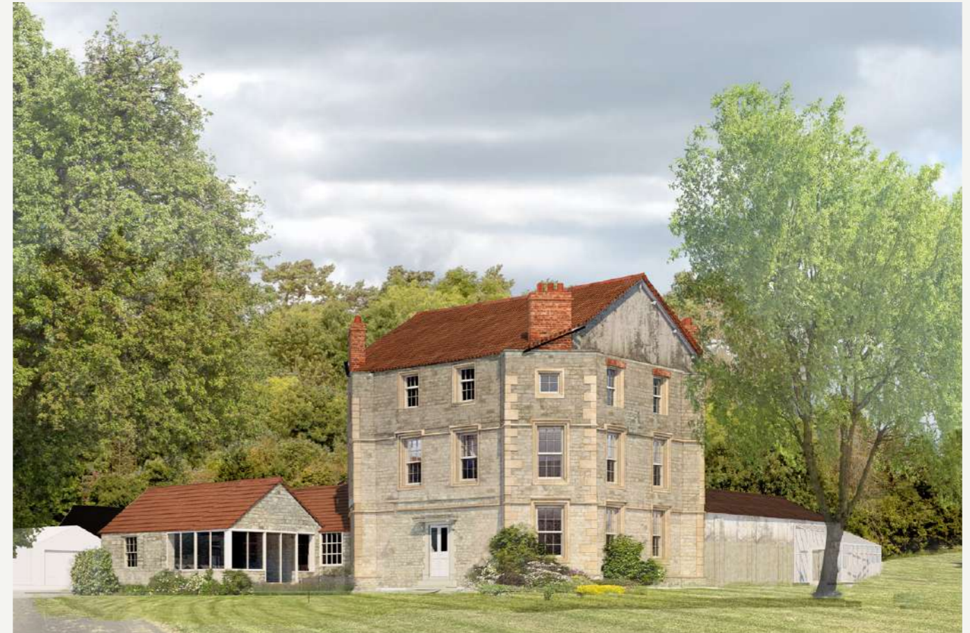
EXISTING SOUTH WEST VIEW
