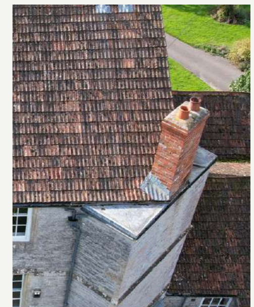
AWKWARD CHIMNEY AND GUTTER JUNCTIONS ARE UNSIGHTLY AND HAVE RESULTED IN WATER INGRESS DAMAGING HISTORIC FABRIC.
