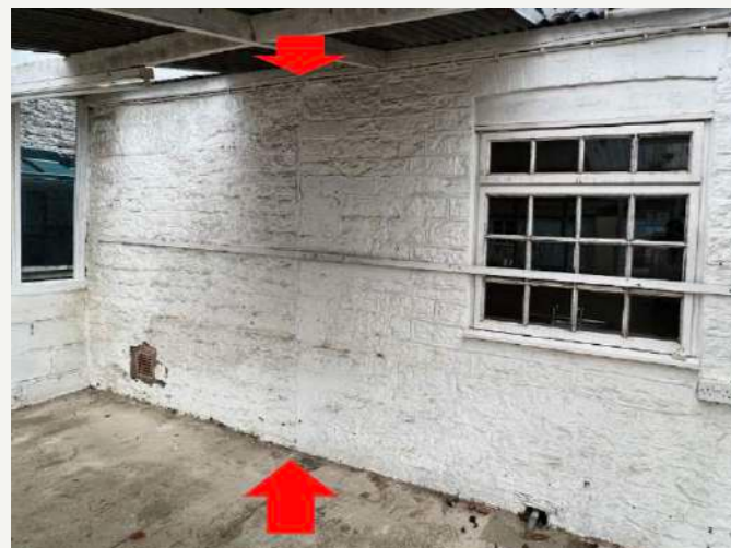
JOINT LINE SHOWING LATER ADDITION OF KITCHEN LEAN TO
