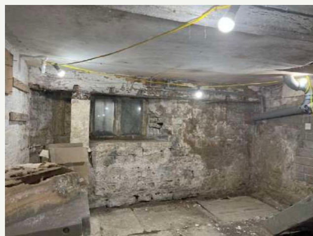
BASEMENT TO BE LEFT IN ITS CURRENT SITUATION
