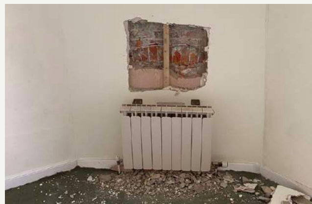
BLOCKED UP FLUES DISCOVERED IN THE CORNER OF EACH OF THE SOUTH BEDROOMS
