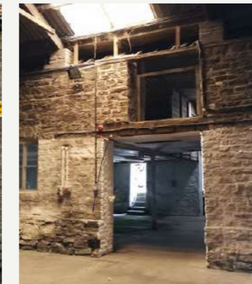
F EXISTING PAIR OF OPENINGS TO BE CONSOLIDATED AS NEW DOUBLE HEIGHT GLAZED OPENING WITH EXTERNAL SHUTTERS
