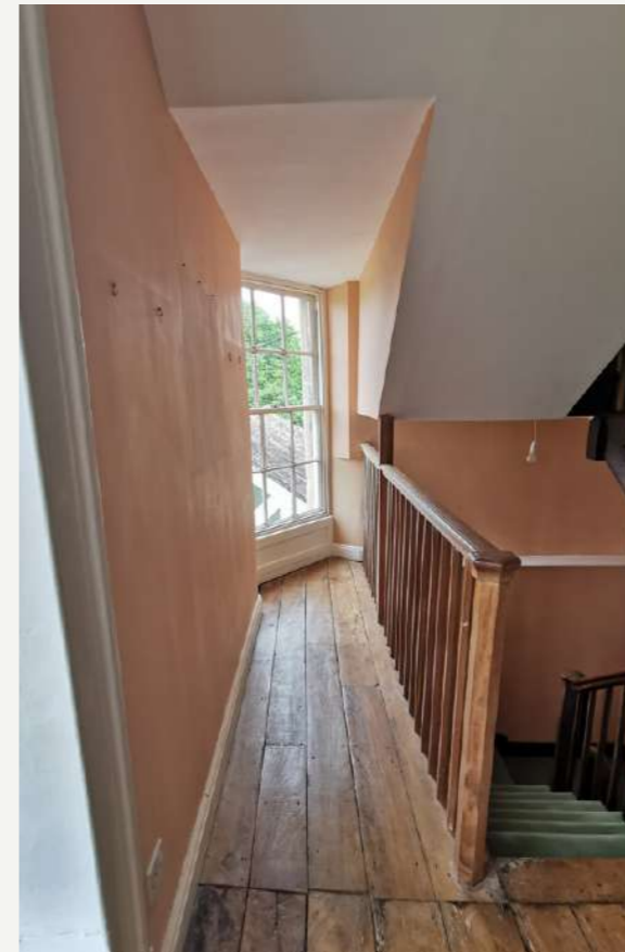
18TH CENTURY WINDOW HEMMED IN BY THE 19 CENTURY LANDING
