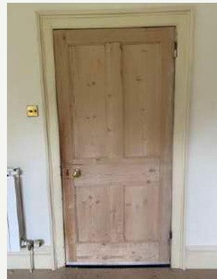
19 CENTURY JOINERY TO BE RETAINED
