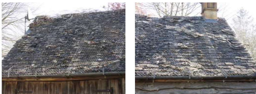
Figs. 5 & 6 Ridges and roof tiles to the front
