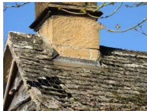
Figs. 9 & 10 Tightly moulded lead flashing
