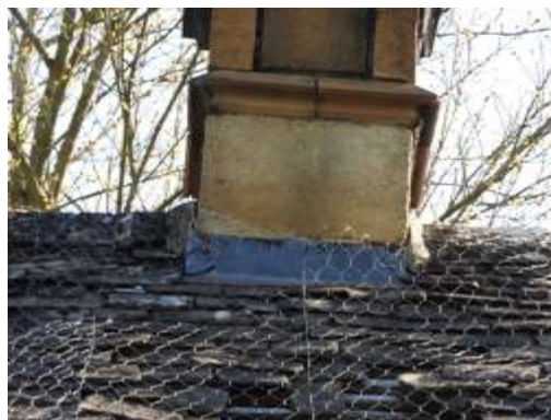
Figs. 9 & 10 Tightly moulded lead flashing
