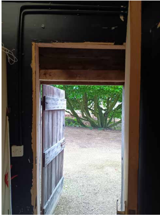
3.10 Detail of modern internal finishes in garage (DIA)
