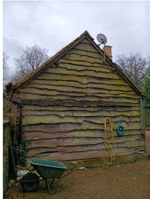
3.4 North elevation of the garage (DIA)
