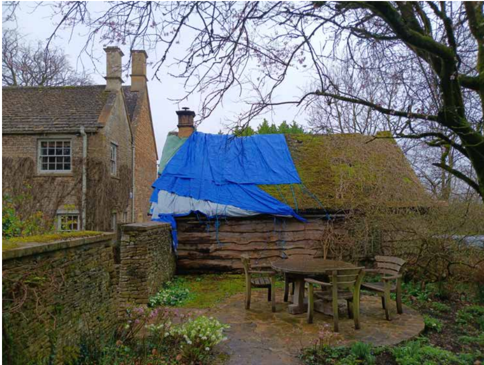
3.5 East elevation of garage (DIA)
