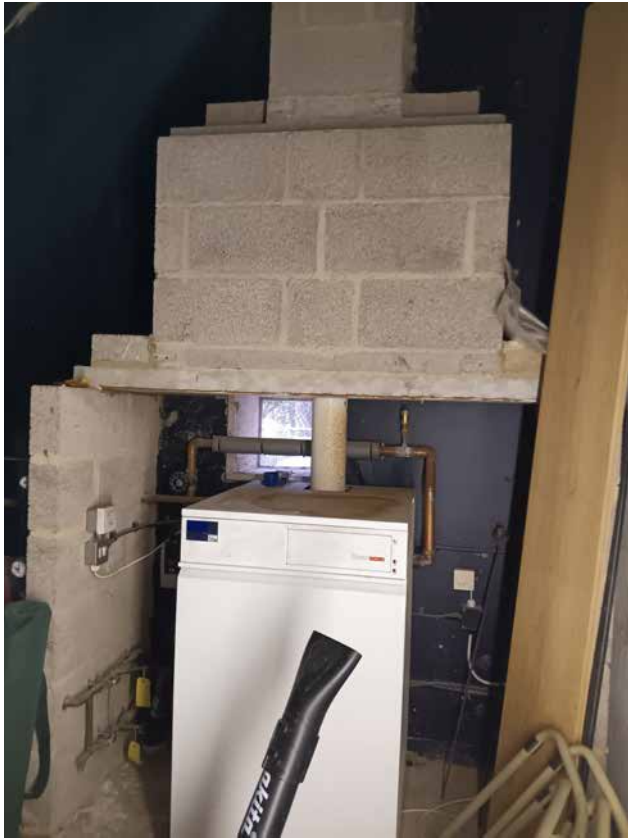
3.12 Detail of blockwork chimney stack of boiler in garage (DIA)
