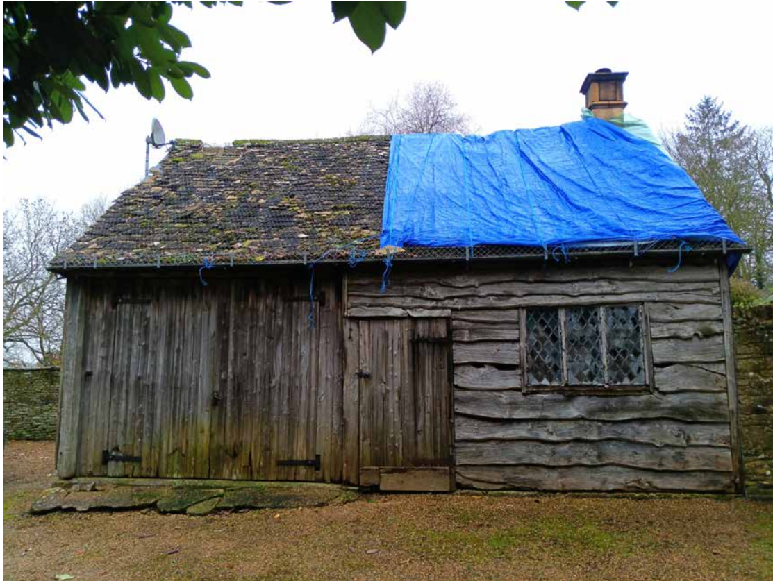
3.3 West elevation of the garage (DIA)
