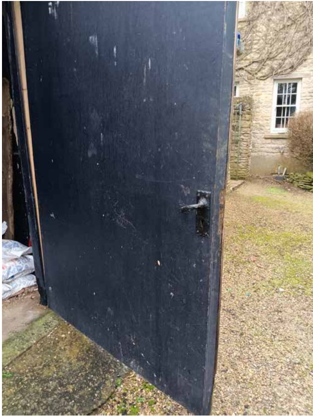
3.9 Detail of modern door (DIA)
