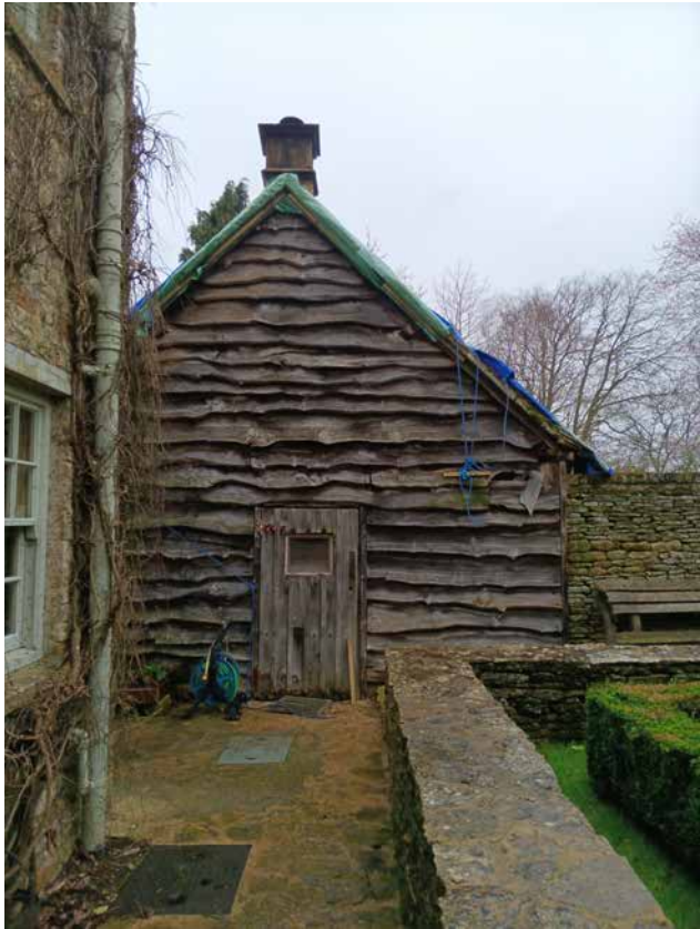
3.7 South elevation of garage (DIA)
