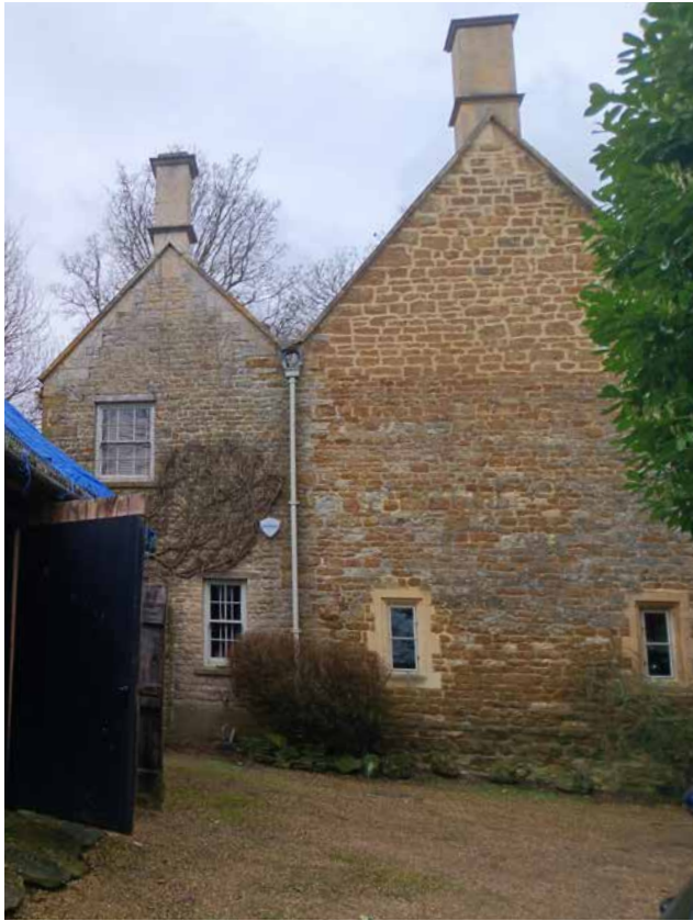
3.1 North elevation of Dower House, with garage to left (DIA)
