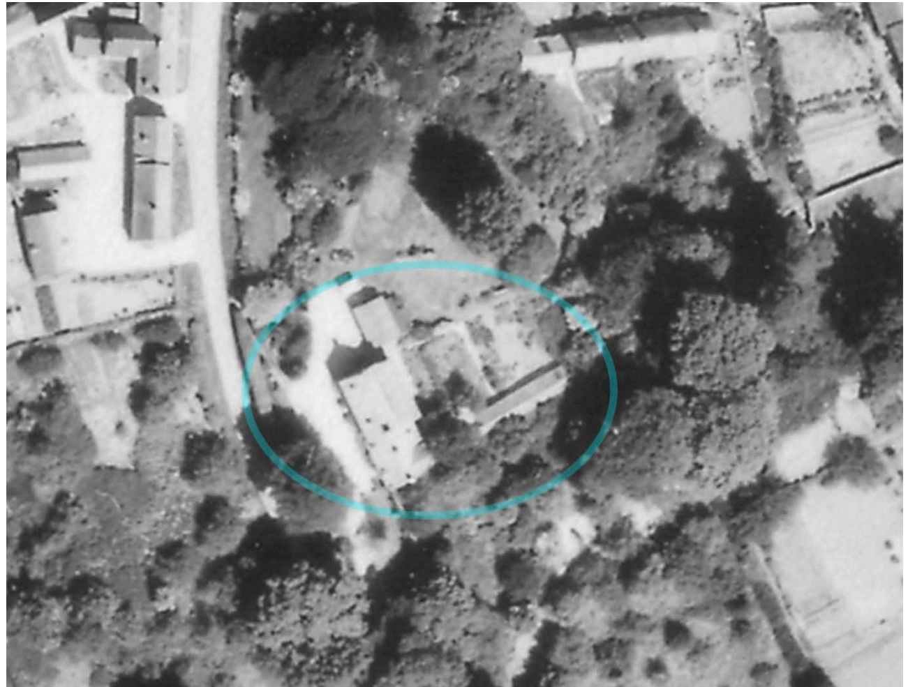
2.5 1961 aerial map showing new north garage set back from the west front of the house (OHC, POX0451726)
