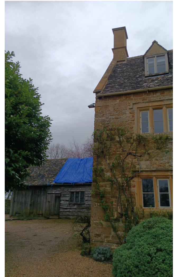
The existing shed set back from the Dower House
