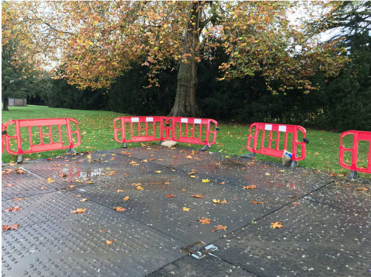
Photo 2. An example of heavy-duty ground protection.
