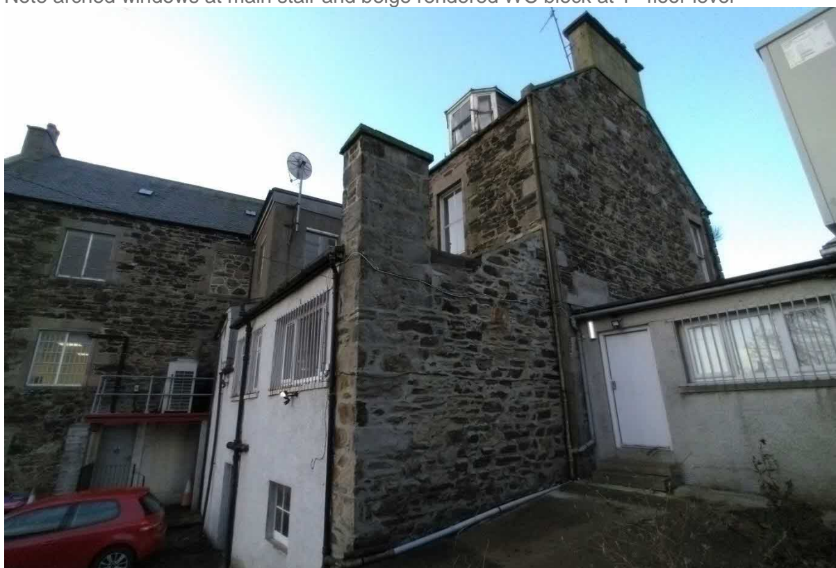
Photograph 5: North / Side Elevation facing Banff Castle + Castle Gardens
