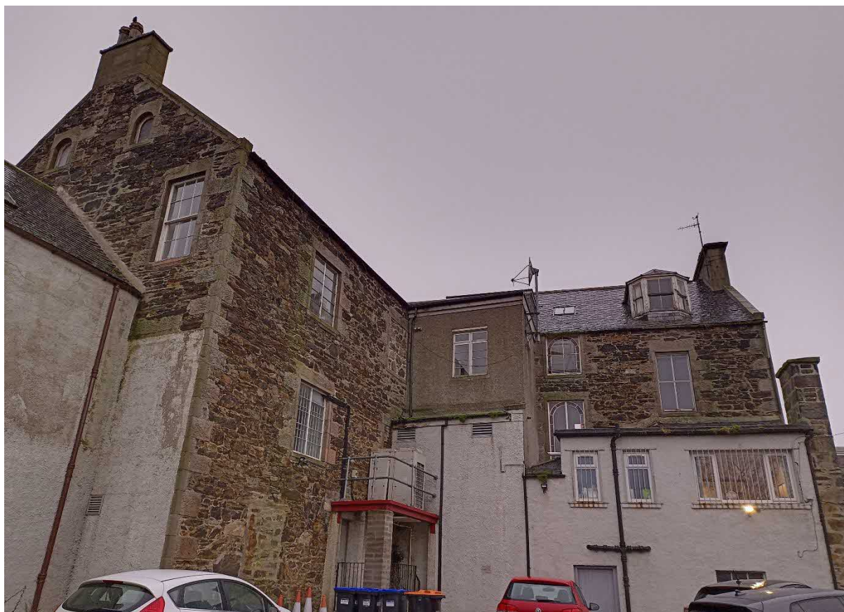
Photograph 4: East / Rear / Old Castle Gate Elevation, Note arched windows at main stair and beige rendered WC block at 1 st floor level
