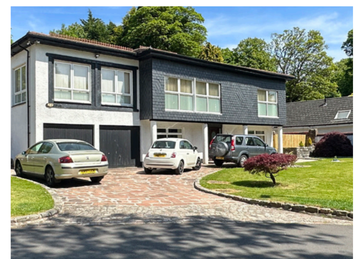
The Paddock development, with contrasting materials to ground and first floor.
