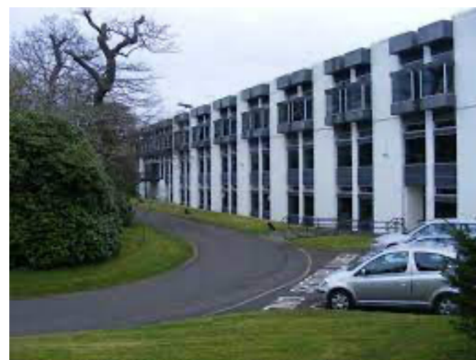
Attached 1960s office building
