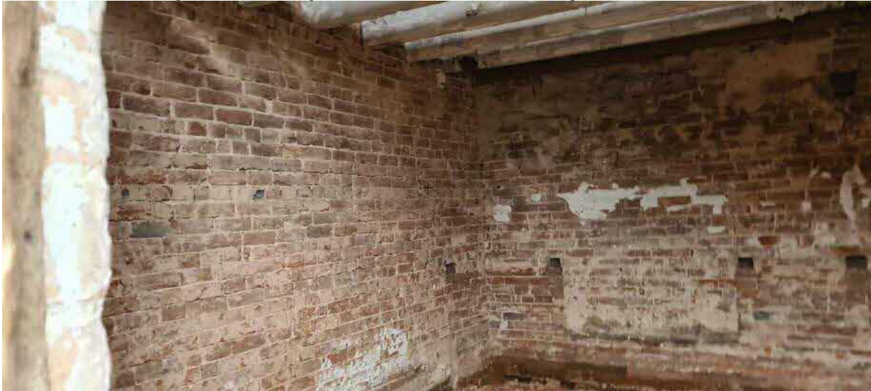
Figure 13 –Existing internal brickwork to be made good and insulated
