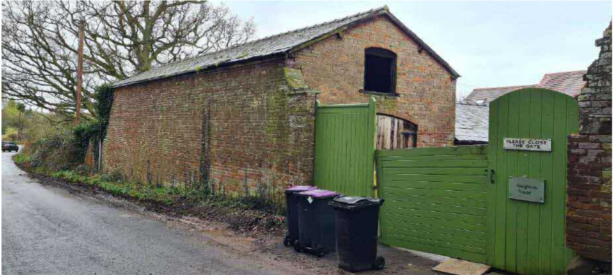
Southern elevation (taken from adjacent public highway)
