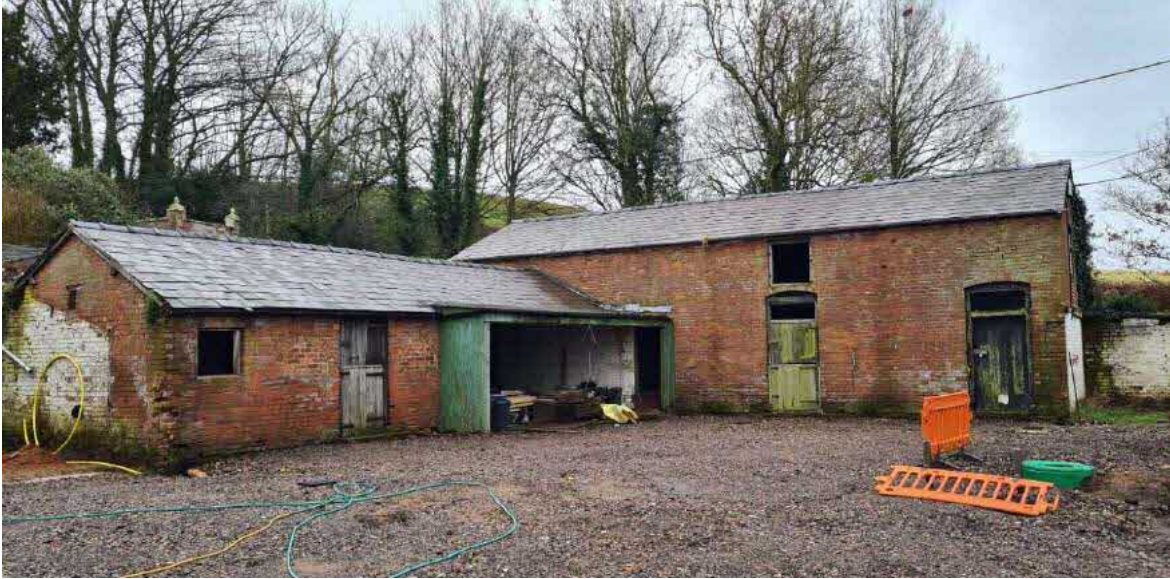
Looking southward from adjacent courtyard
