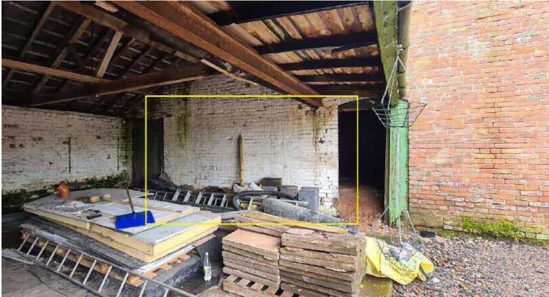
Figure 16 –Section of internal wall to be removed
