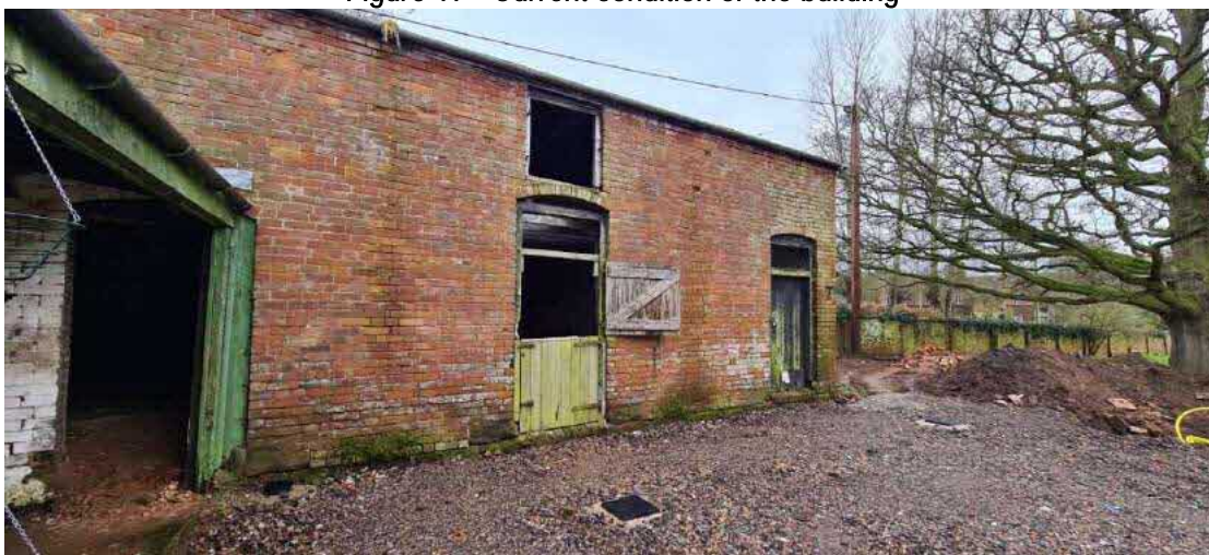
Figure 17 –Current condition of the building
