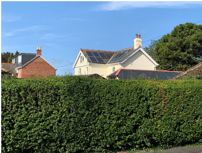
Image 01 - View NW from King's Road showing existing roof
