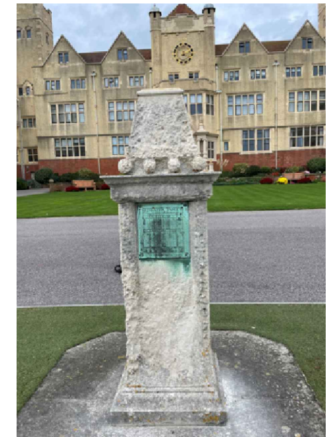
Existing structure, photo taken Oct 31st 2022.
