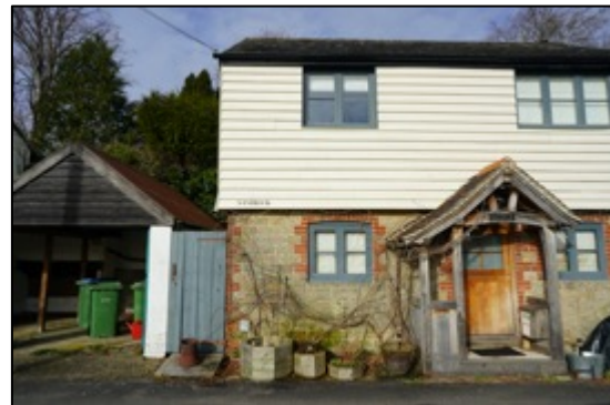
Photo 4: Southern elevation of building B1, facing north.
