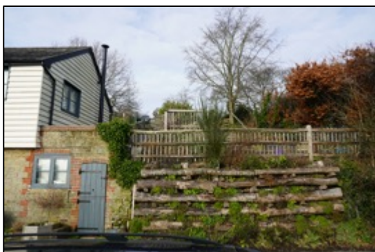
Photo 5: Southern aspect of the Site, showing the timber retaining wall.
