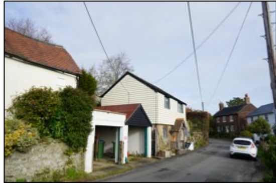
Photo 2: Western elevation of the building B1, facing east.
