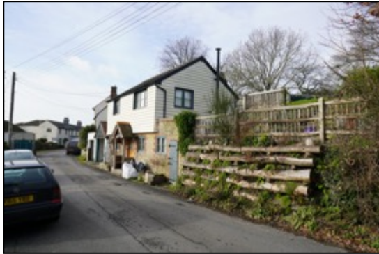
Photo 1: Eastern elevation of the building B1, facing west, showing the retaining wall in the foreground.
