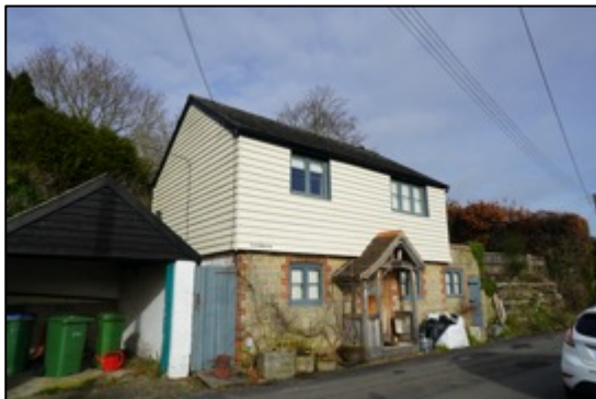
Photo 3: South-western elevation of the building B1, facing east.
