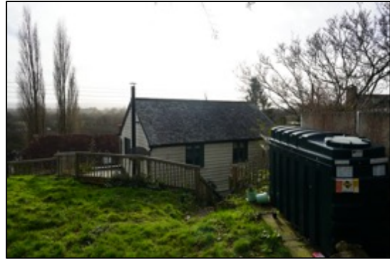
Photo 8: Northern aspect of the Site, facing south, showing the poor semi-improved grassland and building B1 in the background.
