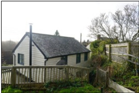
Photo 10: Northern elevation of building B1, facing west.
