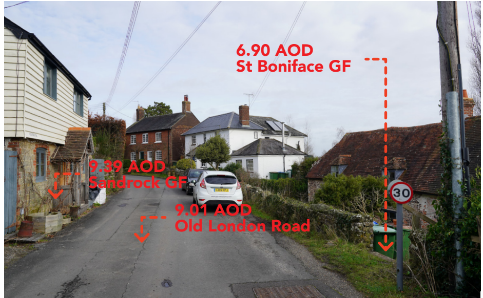
Properties to the south of Old London Road are significantly lower than those to the north.
