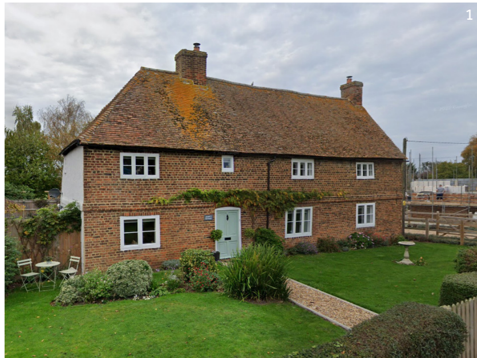
Lockett Cottage | Notice the 4-Panel door, brick band course separating the floors, and the hipped gable end.
