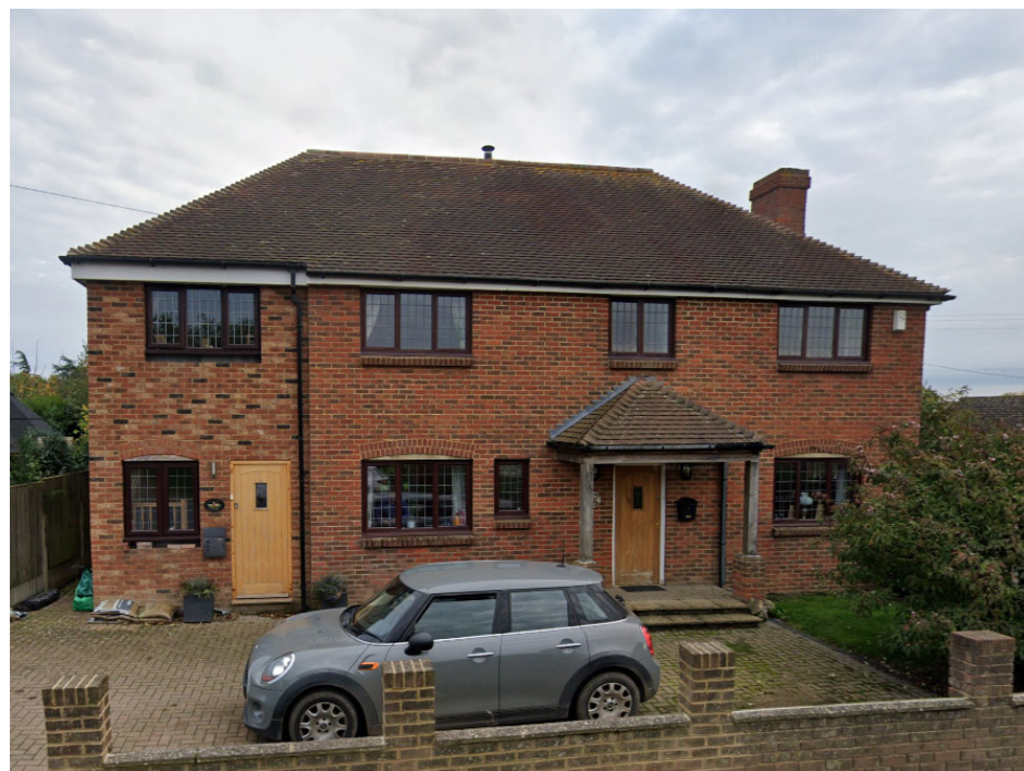
New build | Notice the 2 off-centre farm-style 4-panel doors with central window, the brick soldier course under the windows, and column-supported door canopy.
