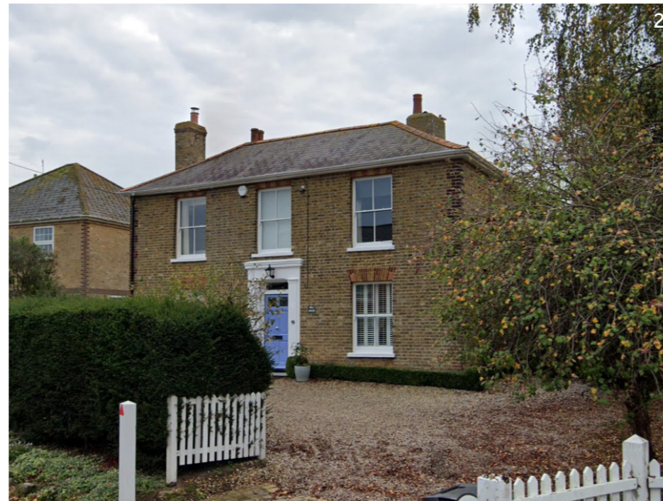
Georgian House | Notice the gauged brick arches above the windows, the 6-Panel door with light and superior decorative pediment.
