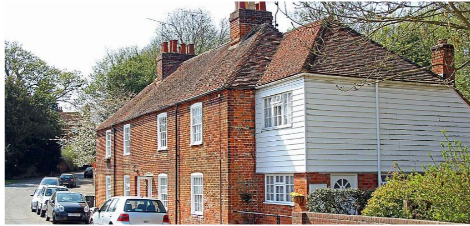
Rural buildings with a mixture of weatherboarding, red stock brick and clay tiles.
