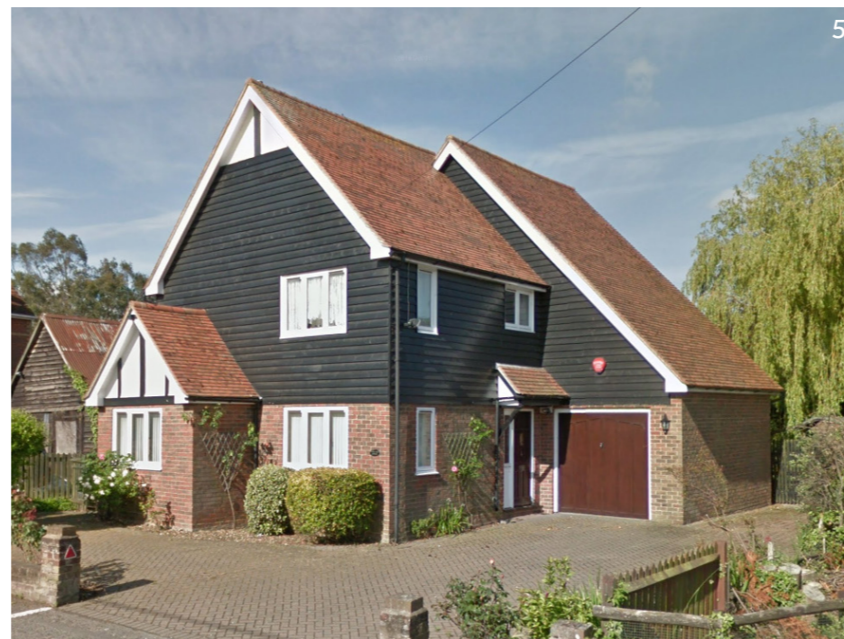
New Build | Notice the Cat-Slide roof, black weatherboarding, and door canopy.
