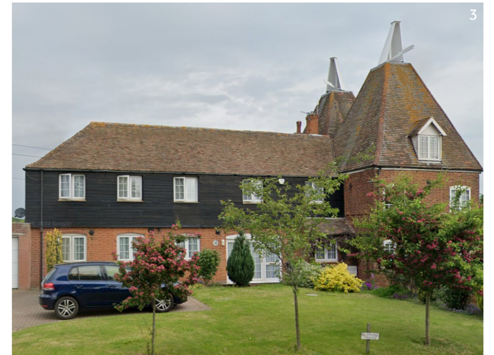
Traditional Oast House | Notice the rubbed brick arches above windows and door, the first floor black weatherboarding and hipped gable end of the roof.
