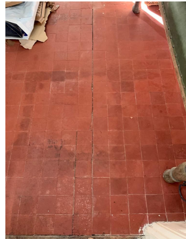
Internal Cracking
