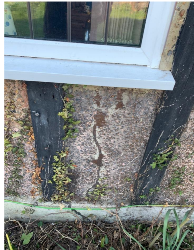
External Cracking
