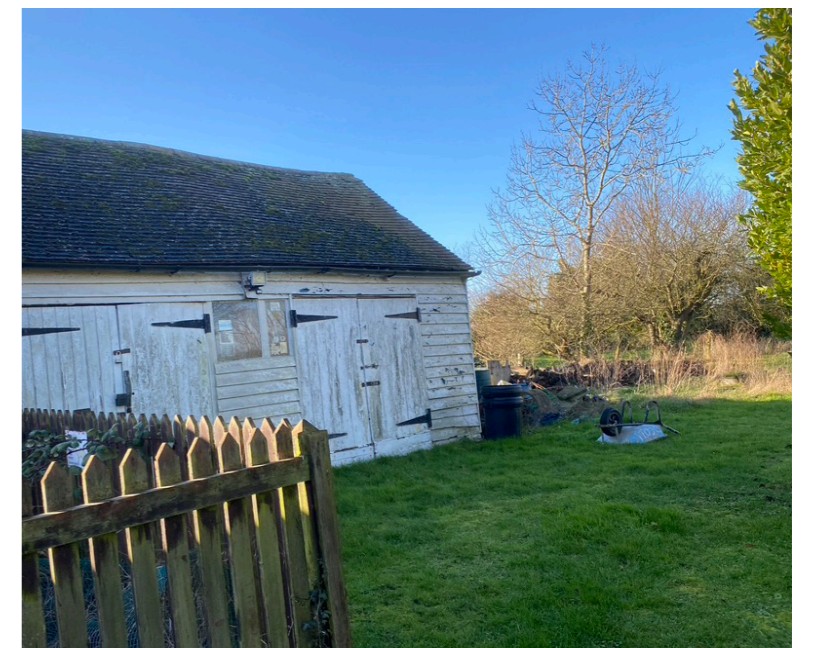
Existing shed structure on the land
