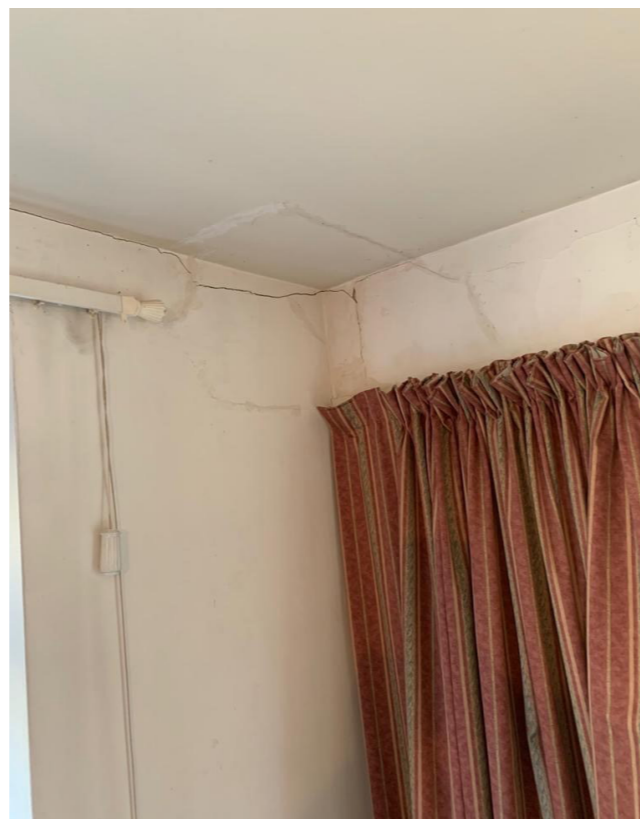
Internal Cracking
