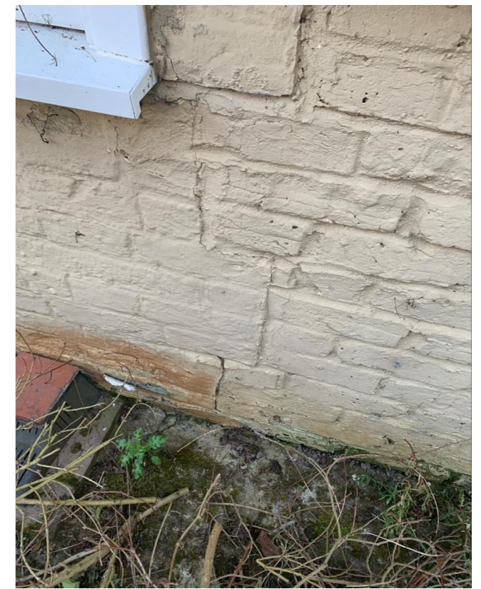
External Cracking
