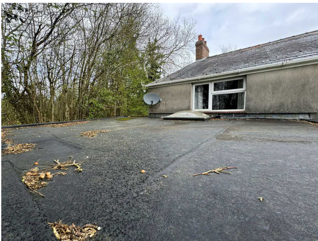
Plate 10. Butyl covering of flat roofed extension.
