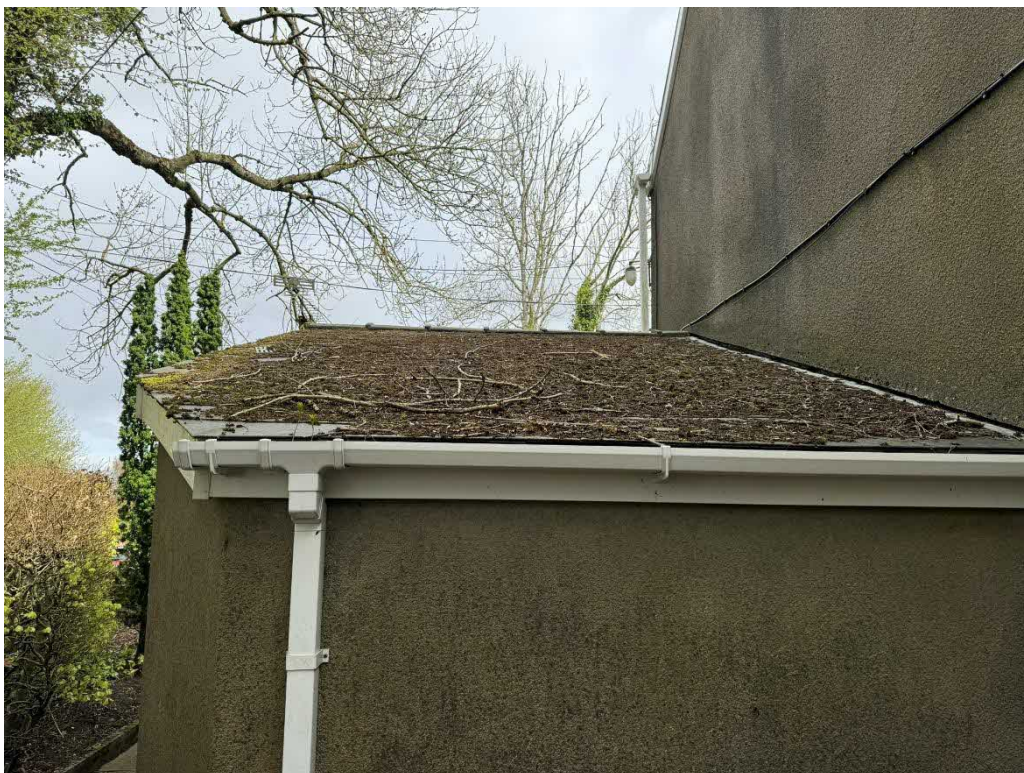
Plate 8. Southern aspect of garage to be removed.
