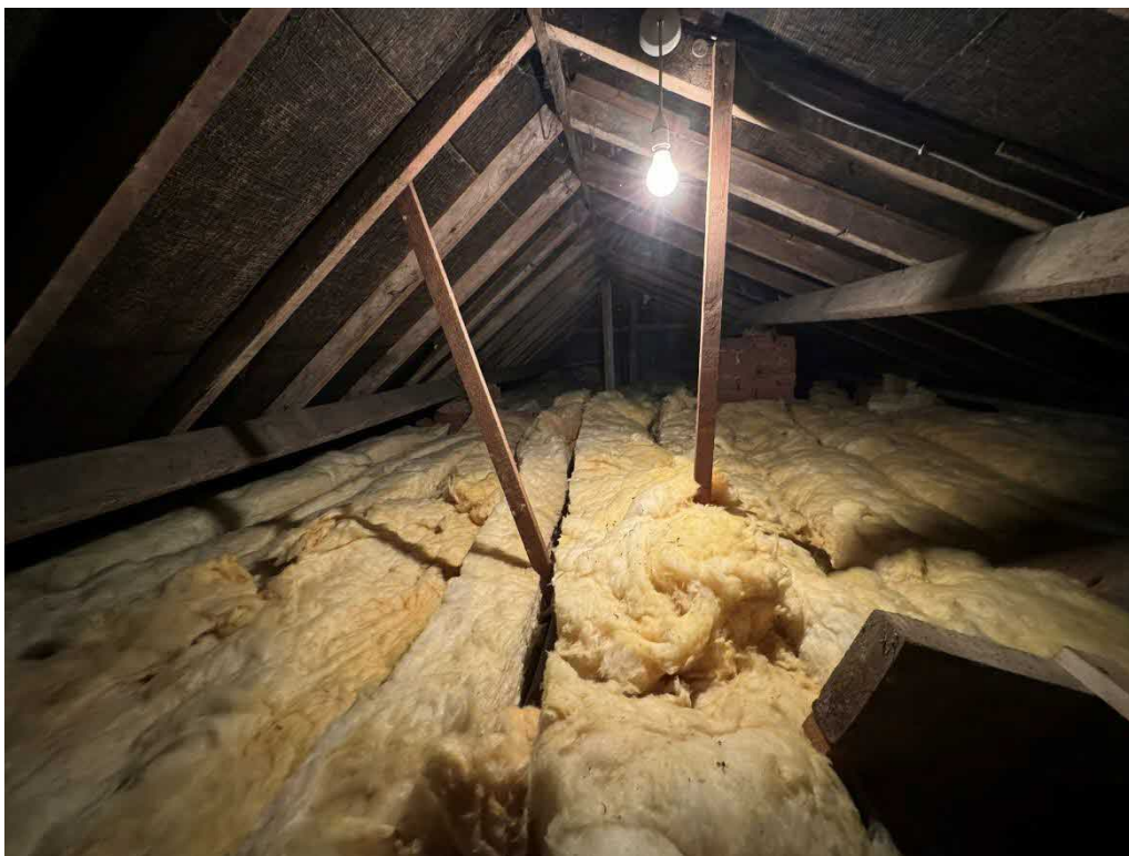
Plate 11. General view of interior roof void.
