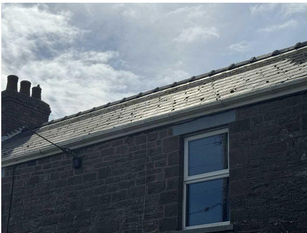
Plate 2. Northern roof aspect.
