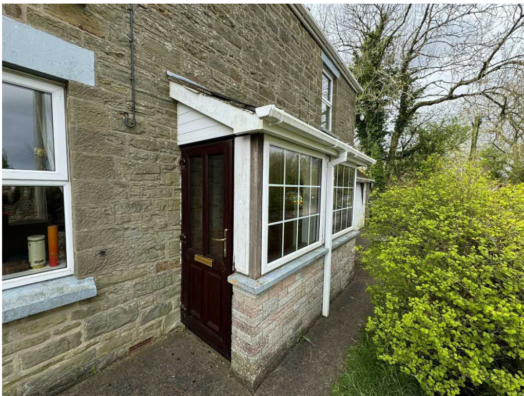
Plate 3. Enclosed porch planned for removal.
