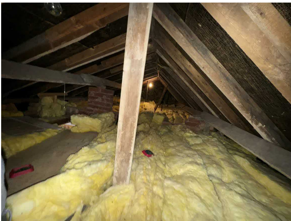
Plate 12. General view of interior roof void.
