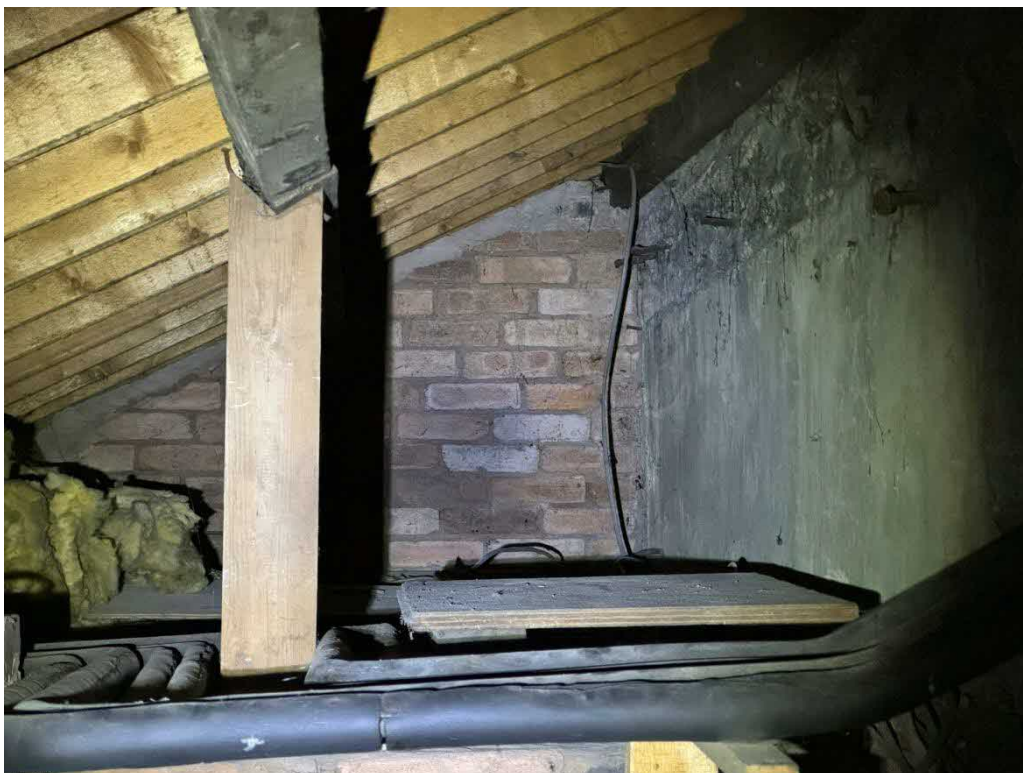
Plate 16. Roof void of eastern extension.
