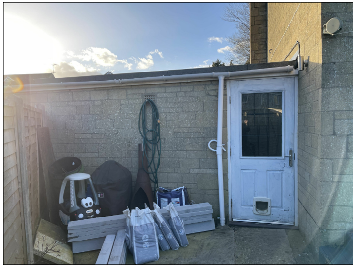
VIEW OF REAR ELEVATION
