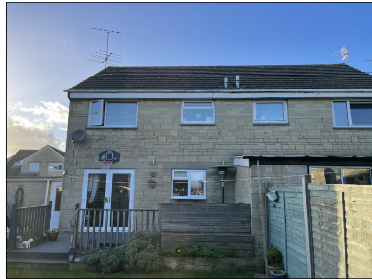
VIEW OF REAR ELEVATION
