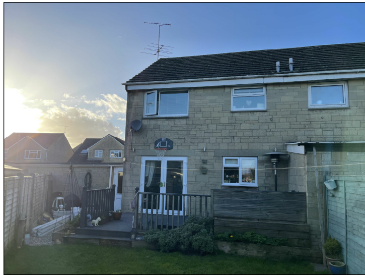
VIEW OF REAR ELEVATION
