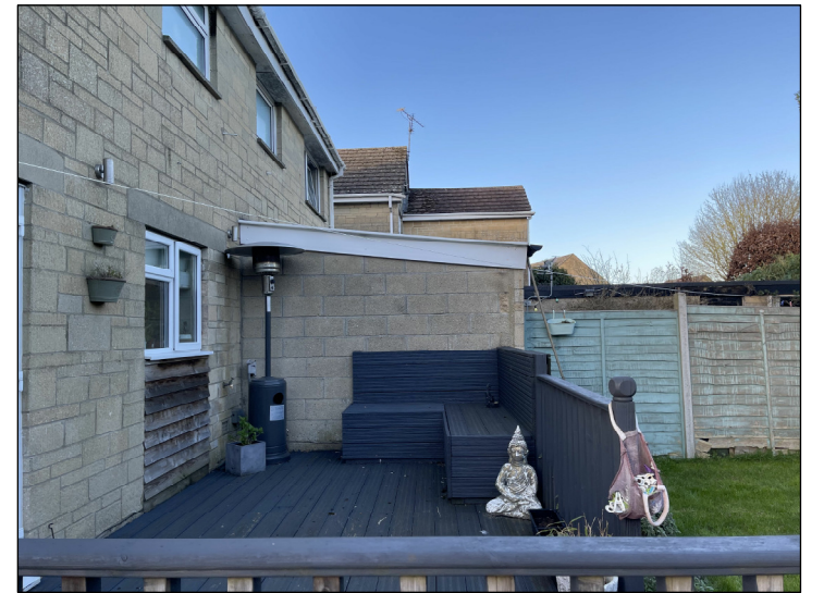
VIEW OF REAR ELEVATION
